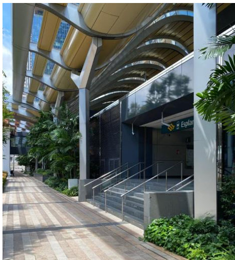
High roof over station entrance attracts rainwater
