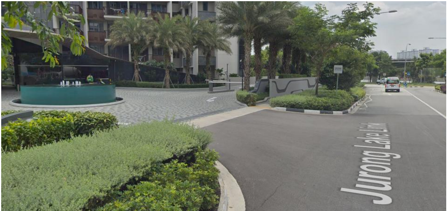
Figure 1: Access of a Residential Drop-Off point located at least 30m from a road junction
