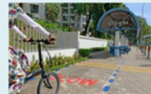
Safety markings to guide riders at bus stops
