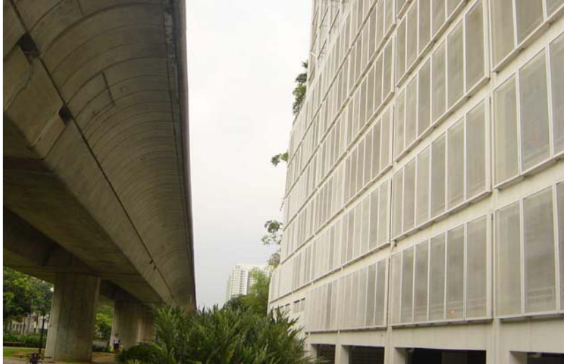
Figure 4-6 A multi-storey car park with façade opening facing the viaduct is provided with a protective screen
