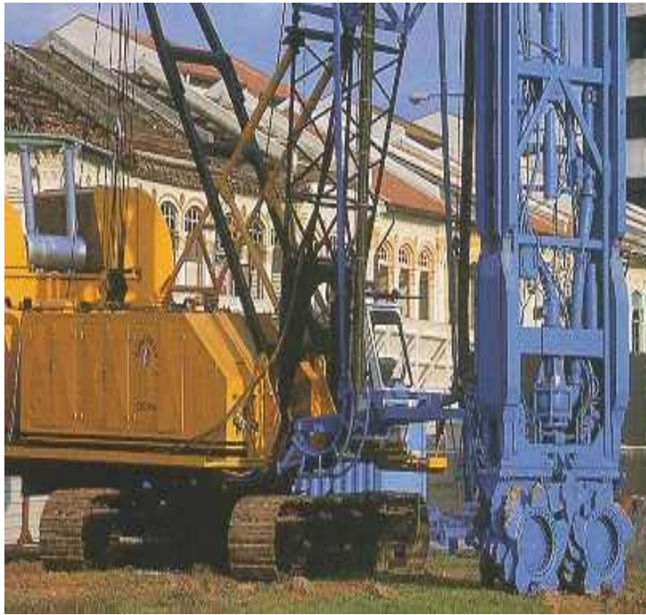
Figure 3-6 View of a hydrofraise machine
