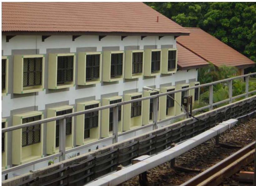
Figure 4-7 A multi-storey car park with façade opening facing the viaduct is provided with a protective screen
