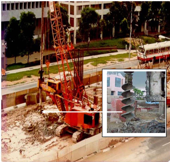
Figure 3-3 Pile installation by augering method
