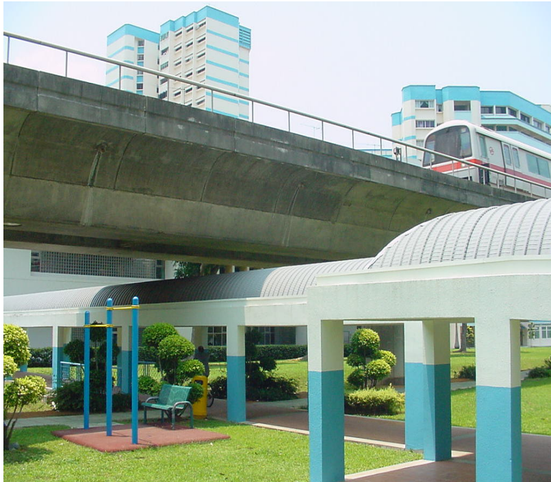
Figure 4-21 Land below the viaduct can be used to locate a linkway
