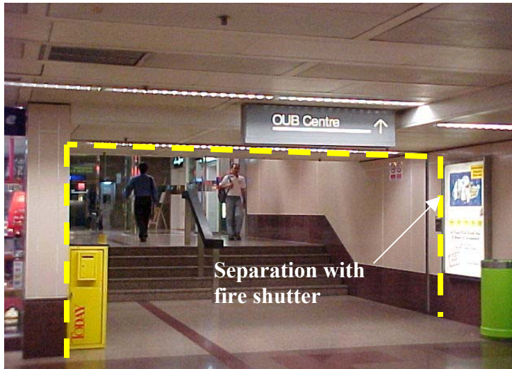
Figure 4-39 Building linked to RTS station
