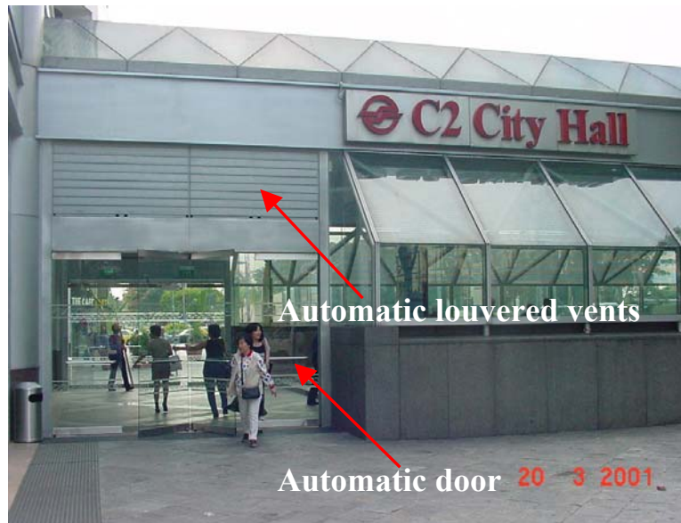
Figure 4-37 View of an enclosed entrance at RTS station
