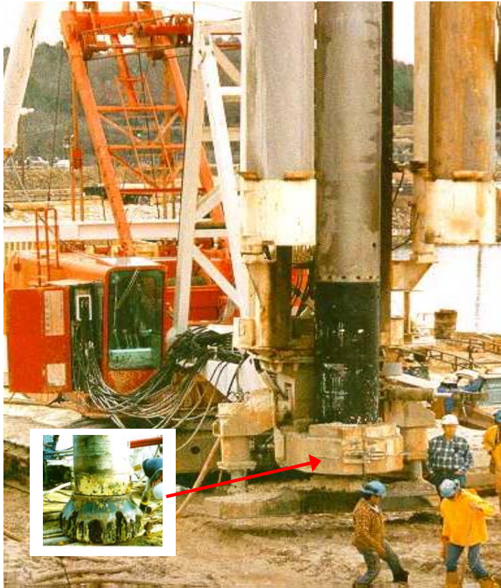
Figure 3-7 Pile installation by down-the-hole drilling technique
