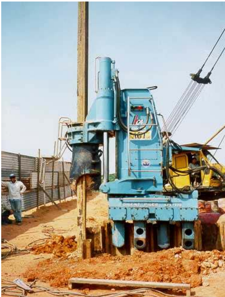
Figure 3-5 Sheetpile installation by a silent piler
