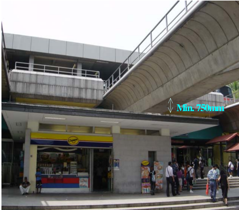
Figure 4-13 A convenience store located under the viaduct
