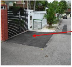
Top of culvert shall be in concrete finish to facilitate road resurfacing works and for pedestrian connectivity
