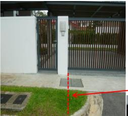
Turning kerb is to be inline with gate post to prevent vehicles from colliding with the gate post or mounting over the kerb and road sidetable
