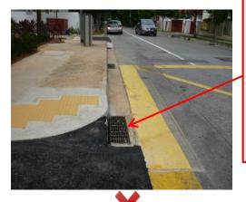
Drop in-let chamber shall be provided at the tangent point of the turning kerb to ensure surface water runoff to be discharged at lowest point, to prevent water stagnation.
