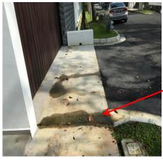
Top of culvert shall be levelled correctly to prevent water stagnation
