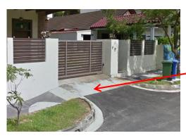
Top of culvert shall be flat to ensure safe path for pedestrians to cross entrances
