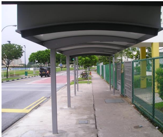
Type 1PC - Single pole curve roof
