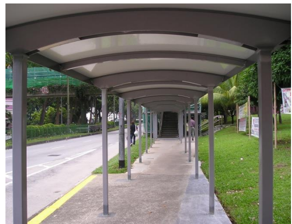
Type 2PC - Double pole curve roof
