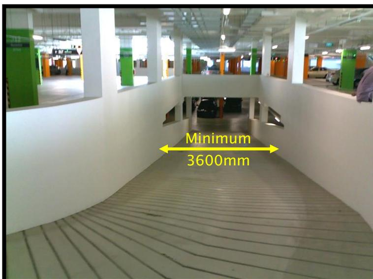
Fig 2.1.3d Example of a single, straight lane
