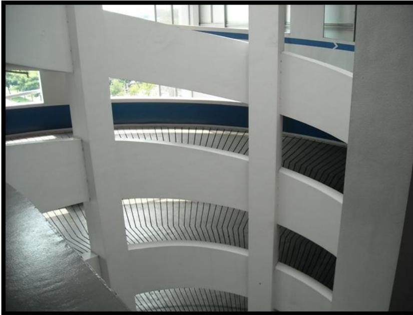
Fig. 4.10a Continuous spiral ramps shall be limited to 4-stories
