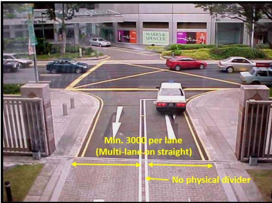
Fig 2.1.3e Example of a straight, multi-lane
