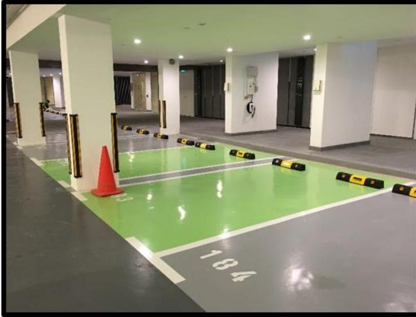
Fig. 4.6b Demarcation of parking lots using different colour tone and serially numbered
