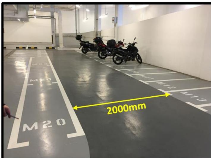
Fig 2.3.1c Parking aisle for motor-cycle
