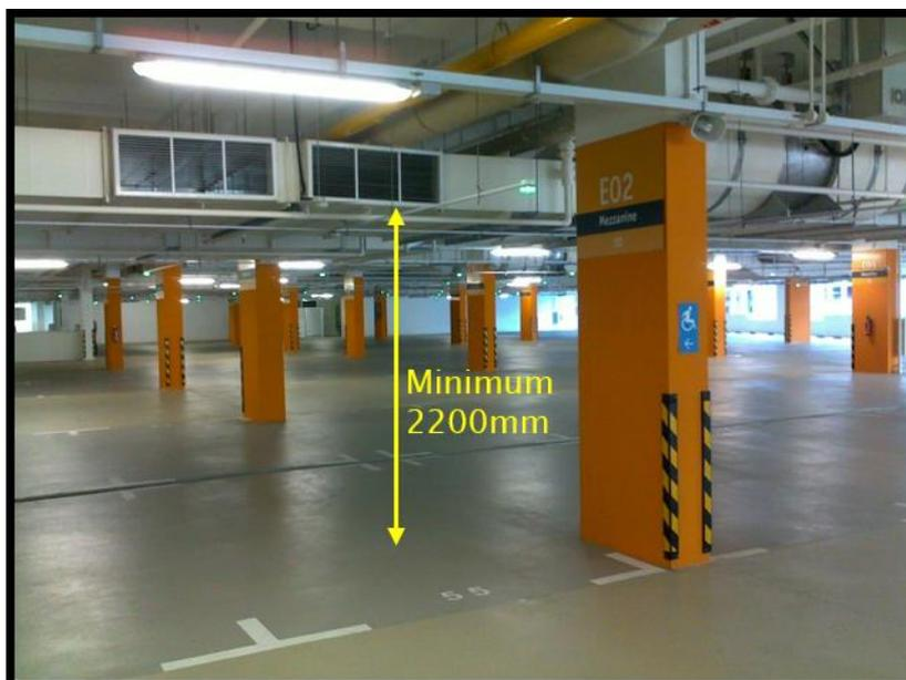
Fig 2.1.5b Example of minimum headroom clearance
