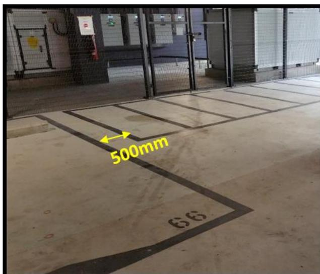
Fig 2.3.1b Example of motor-cycle adjacent to car lot
