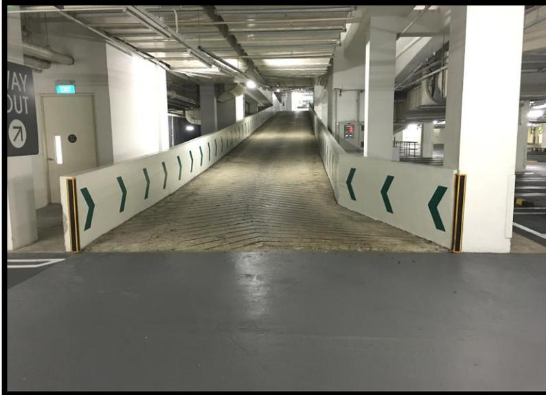
Fig 4.3a Splay corner at bend for better manoeuvring space
