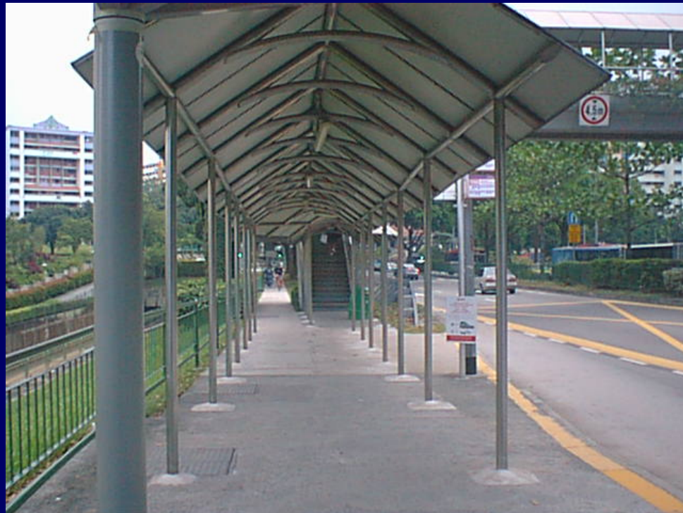
Example of covered linkway with adequate overhang
