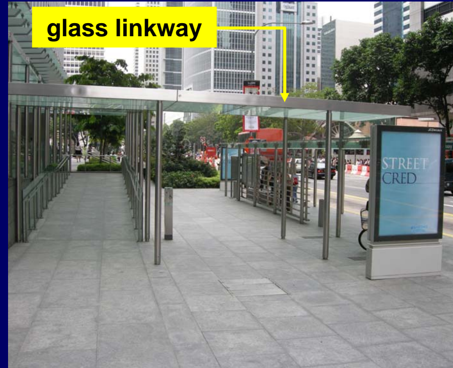
Example of glass linkway where it acts as an extension of the bus shelter
