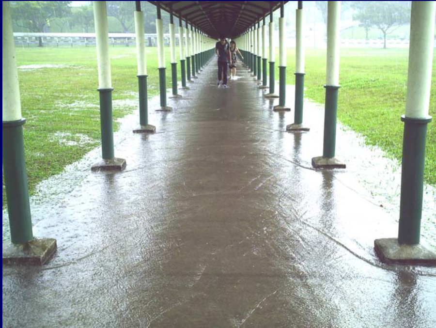
Example of ponding at covered linkway
