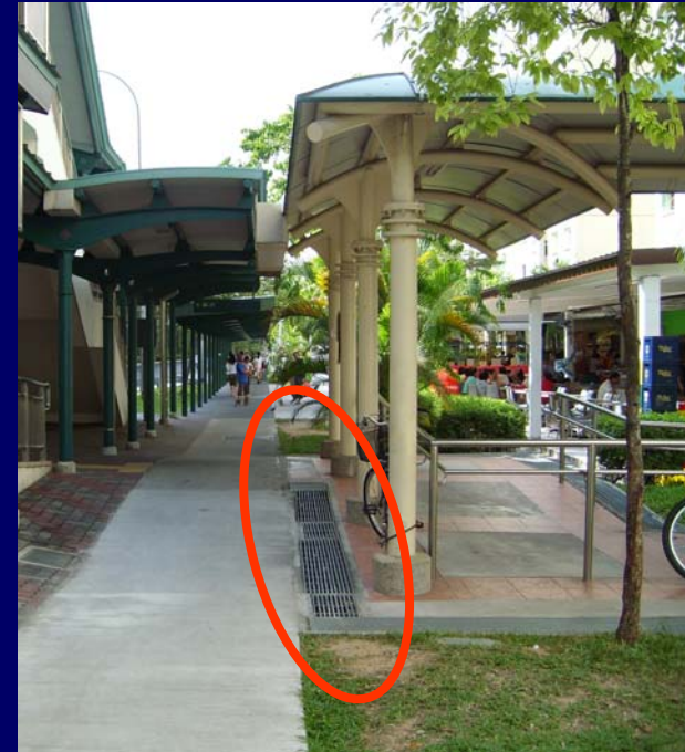
Example of proper drainage measure provided at covered linkway
