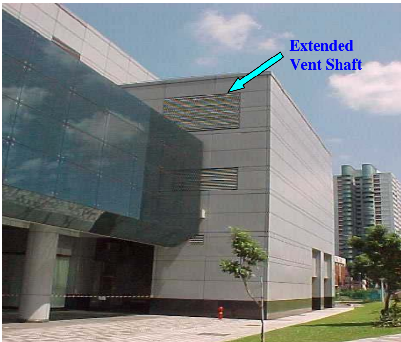
Figure 4-29 Building with RTS ventilation shaft extended from the existing one at ground level
