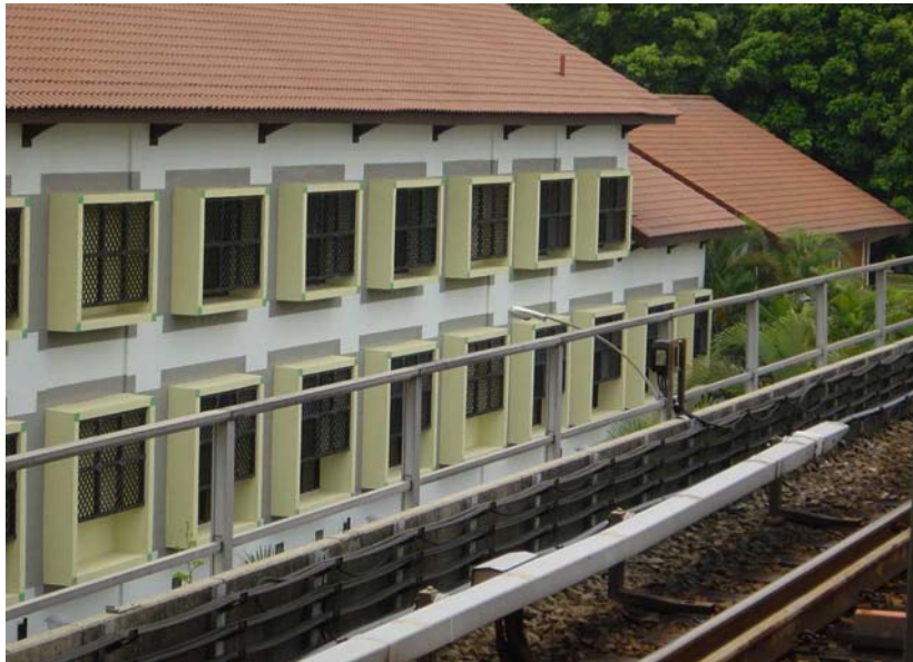
Figure 4-7 A multi-storey car park with façade opening facing the viaduct is provided with a protective screen
