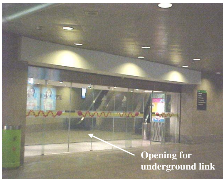
Figure 6-3 An opening created in the wall at concourse level of Bugis Station
