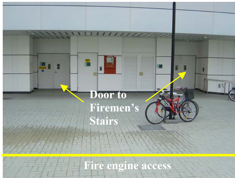
Figure 4-41 The firemen's staircase cum emergency exit at RTS station
