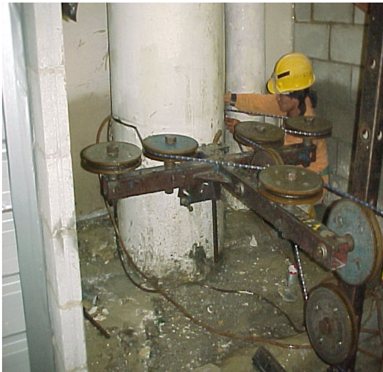
Figure 2-14 Use of a diamond wire saw for cutting station structure helps to minimise vibration and noise levels
