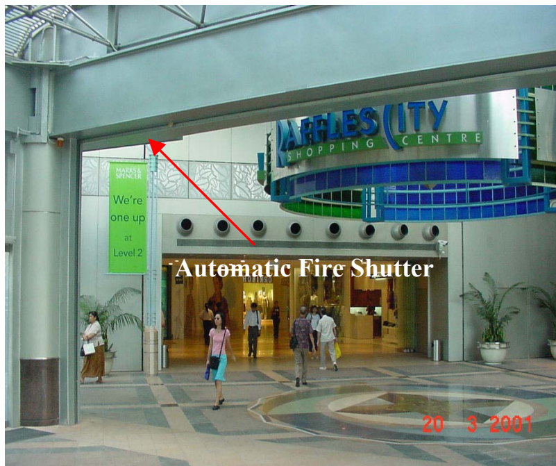
Figure 4-36 An automatic fire shutter at the interface between the commercial development and station entrance
