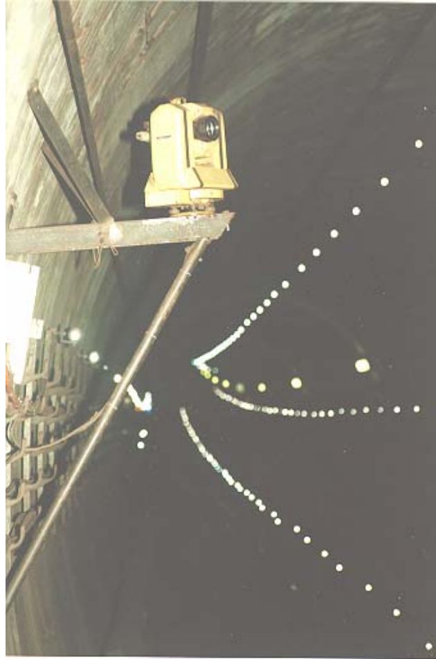
Figure 5-2 Total station in bored tunnel
