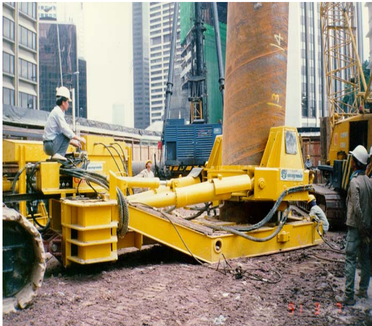
Figure 3-4 Pile installation by oscillatory method
