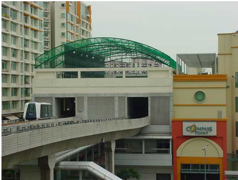
Figure 4-23 View of structures above and around the trainway
