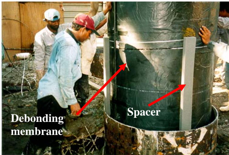
Figure 3-10 Spacer provided to prevent the debonding membranes from any damage during installation
