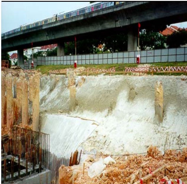
Figure 2-2 Provision of first reserve line demarcation on site
