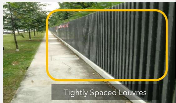
Figure 3.6 - Pedestrian access with Tightly Spaced Louvres
