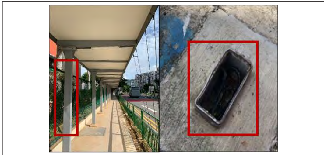
Figure 17: An example of Rectangular Hollow Section (RHS) of Columns Steel Members
