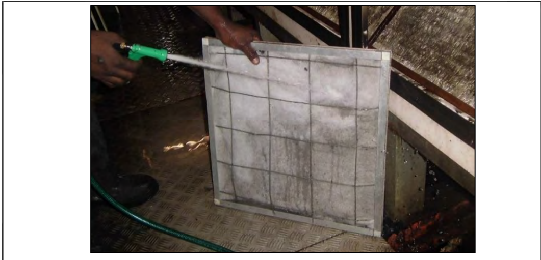
Figure 63: Water Point with Hose for AC Filter Cleaning
