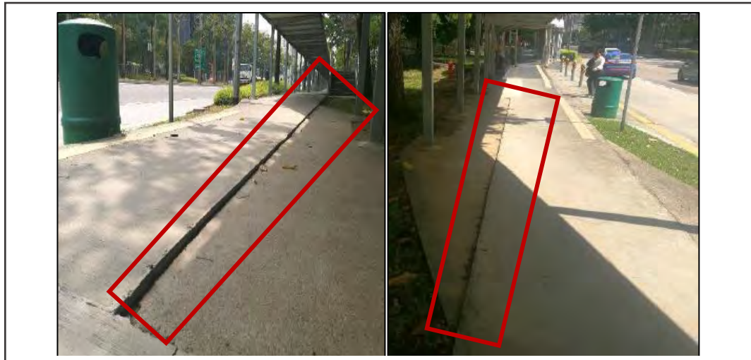
Figure 33: Examples of No Proper Interfacing (i.e. No Dowel Bars Installed) Between the Existing Footpath and New Footpath, Resulting in the Differential Footpath Level
