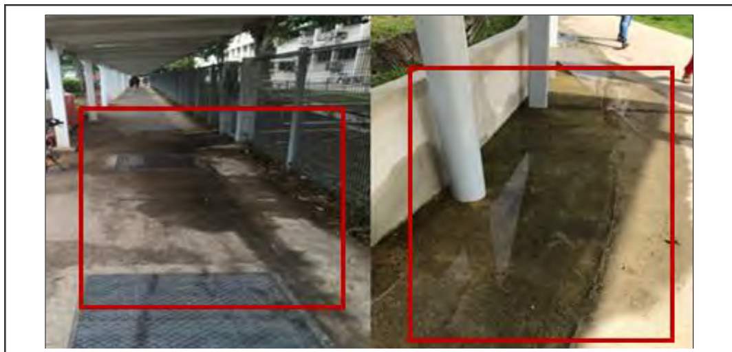
Figure 16: Examples of Water Stagnation on Footpath underneath Covered Linkway Shelter
