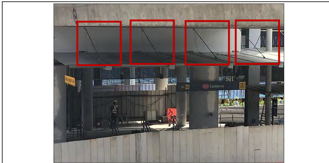
Figure 1: An Example of a Dependent Structure Connected to an Adjacent Structure, a Pick-up Shelter is Structurally Dependent on Adjacent Structure via Tie Rods
