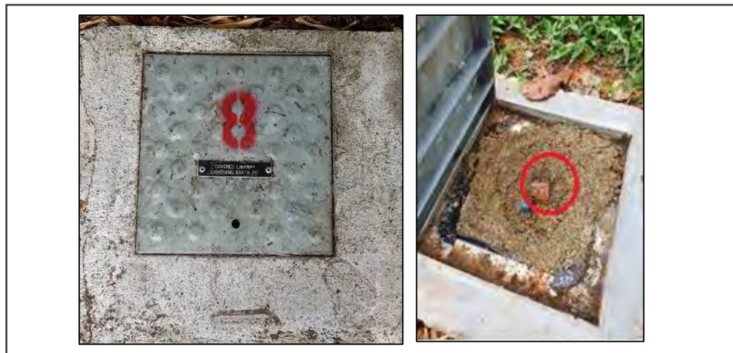
Figure 43: Encase with Concrete and Lightning Rod with Tag
