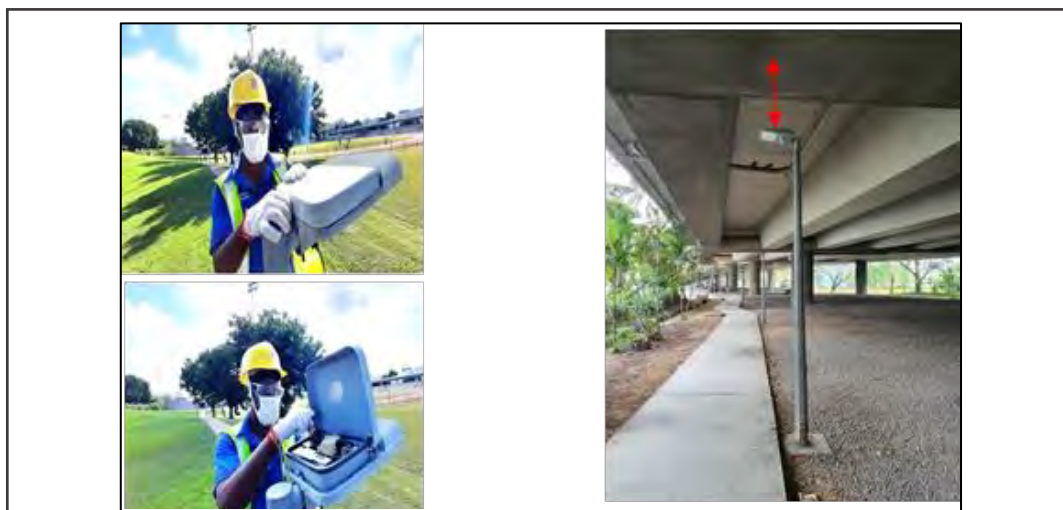
Figure 46: Sufficient Head Space for Top Opening
