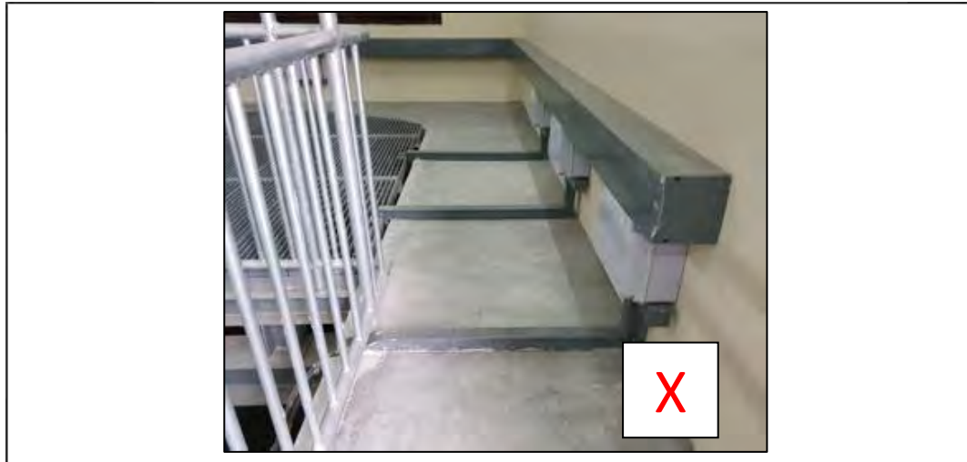
Figure 60: Installations on the Floor are a Tripping Hazard
