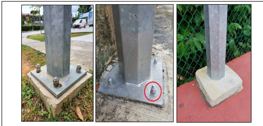
Figure 48: Double Locking Nuts and Haunching of Footing
