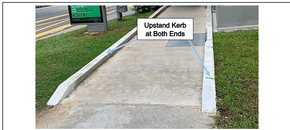
Figure 31: An Example of Footpath with Upstand Kerbs at Both Ends
