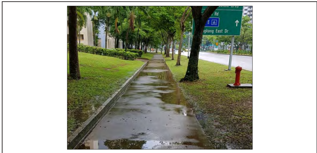
Figure 29: An Example of Adjacent Planting Verge Being Higher than Footpath, Resulting in Water Stagnation
