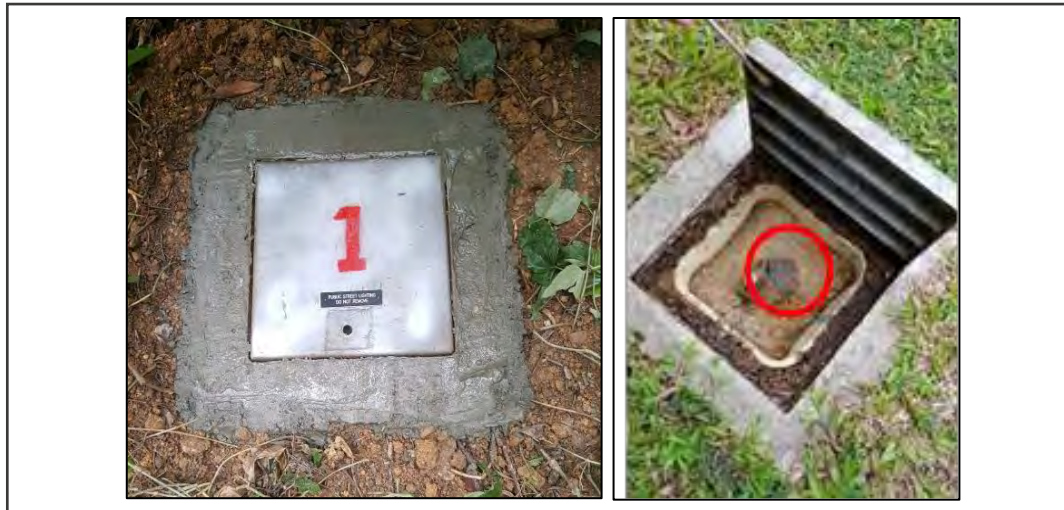
Figure 42: Encase with Concrete and Earthing Rod with Tag
