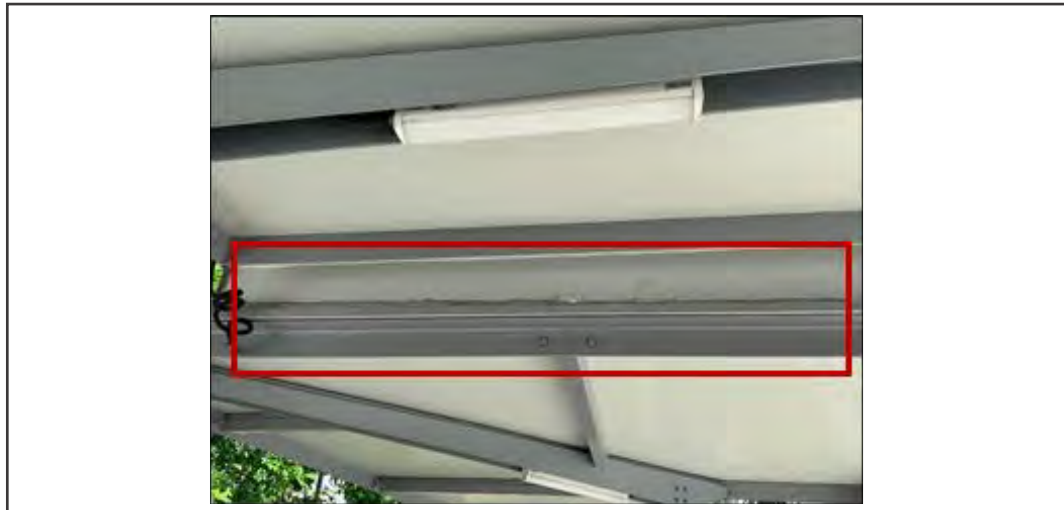
Figure 24: Sealant Applied on Interfacing Element
