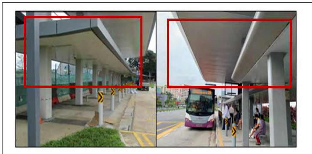
Figure 4: Cladded Roofs of Pick-up Shelter and Bus Stop Shelter are Not Recommended
