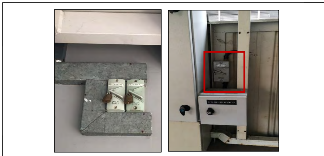
Figure 52: Example of Externally Mounted Power Isolator for CFE System
