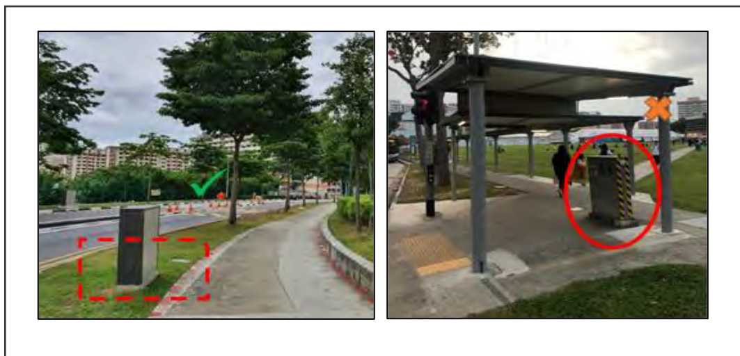
Figure 35: OG Box Position shall Not Block Commuter Movement or be in the Middle of the Walkway
