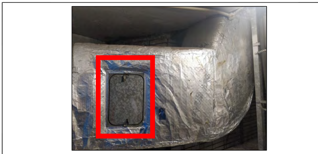
Figure 62: AC Duct Opening
