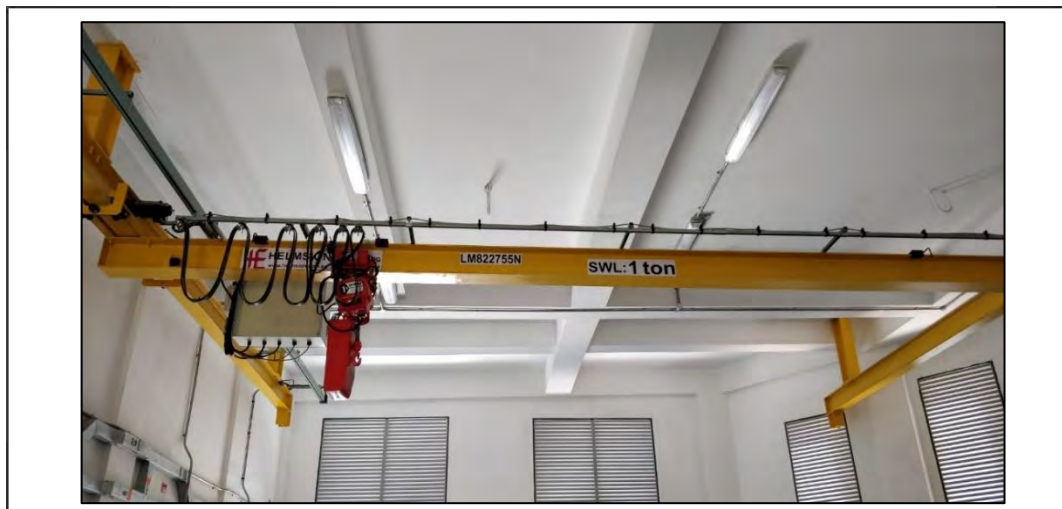
Figure 58: Example of an Overhead Crane for Lifting Pumps
