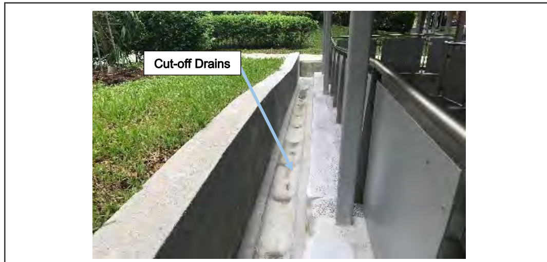
Figure 23: Cut-off Drains Surrounding POB Lift Shaft
