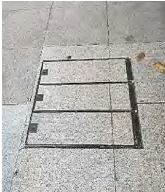
Typical in-filled grating matched with existing floor finishes
