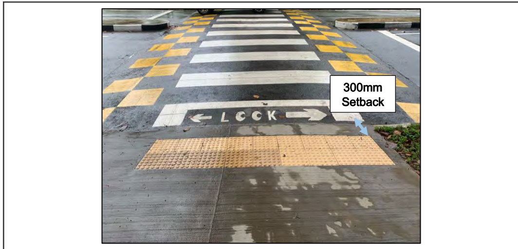
Figure 32: An Example of a 300mm Set back of Tactile Tiles from Footpath Edge
