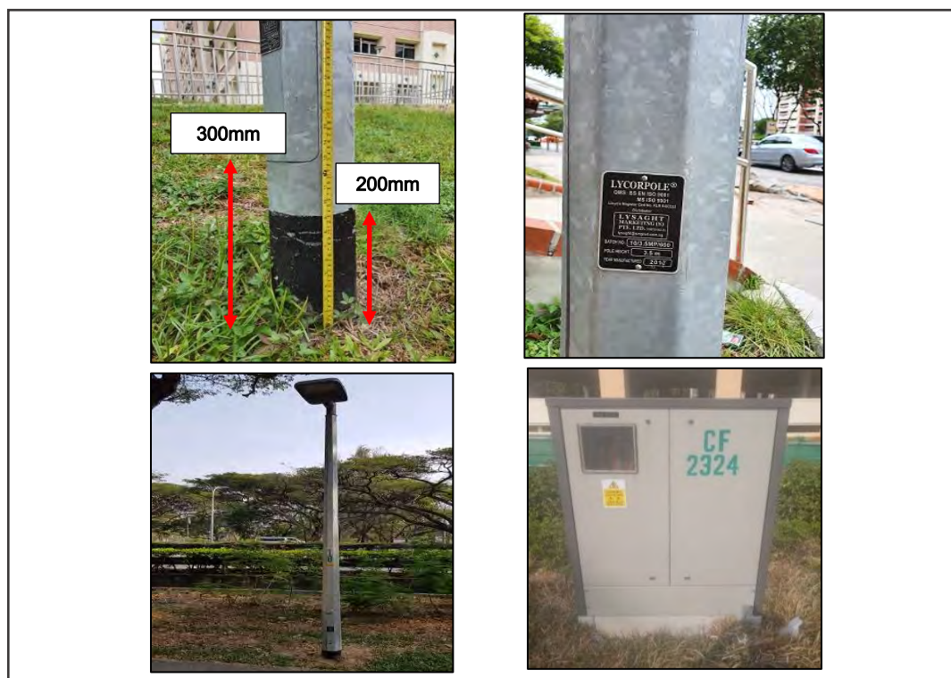
Figure 47: Sufficient Planting Depth, Data Plate and ID
