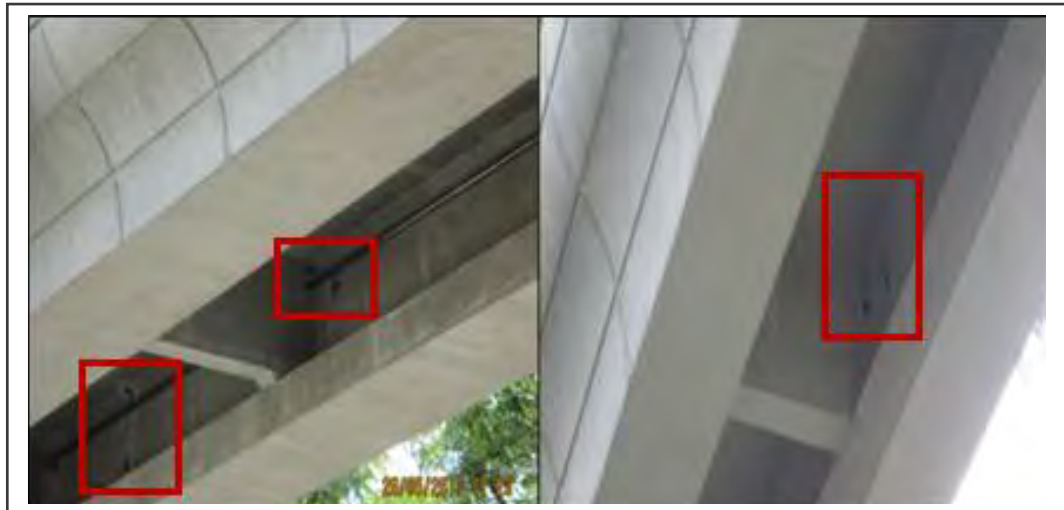
Figure 21: All Unutilised Pre-Designed Holes Shall be Sealed
