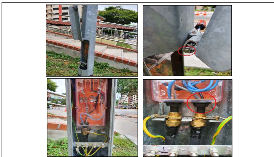
Figure 49: Pole Door Opening, C-clip and Rubber Gasket
