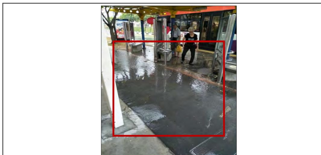
Figure 8: An Example of No Cut-off Drains Behind Bus Stop Shelter, Surface Run-off from Adjacent Higher Grounds Flowing onto Platform underneath Bus Stop Shelter
