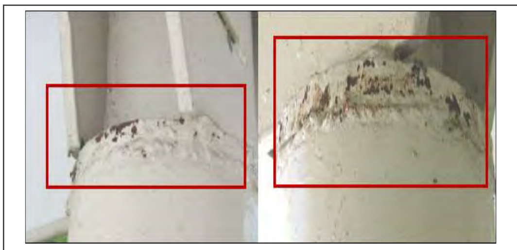
Figure 25: Examples of Corroded Welded Joint Connections at Shelter Roof Members
