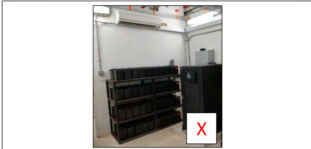
Figure 61: FCU Positioned Directly above Battery Bank
