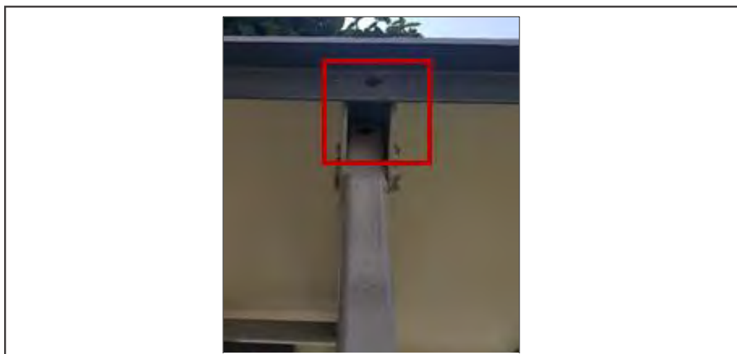
Figure 18: All Unutilised Pre-Designed Holes Shall Be Sealed
