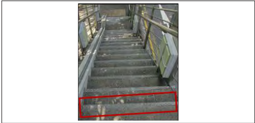
Figure 26: Metal Nosing Tiles (i.e. Steel) are Not Recommended
