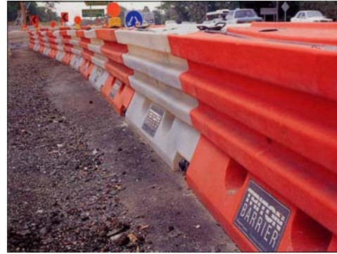
Example of safety barrier that meets NCHRP Report 350 Test Level 2 Crash Test
