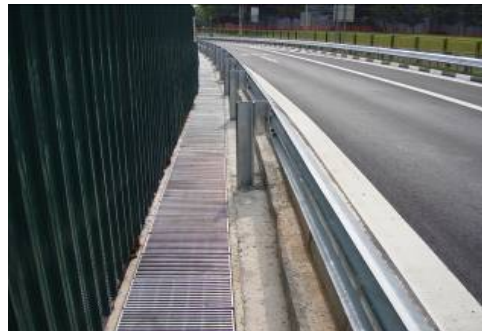
Clear zone provided behind the w-beam VIG
