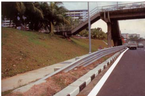
Example of temporary D1 kerbs used in road widening
