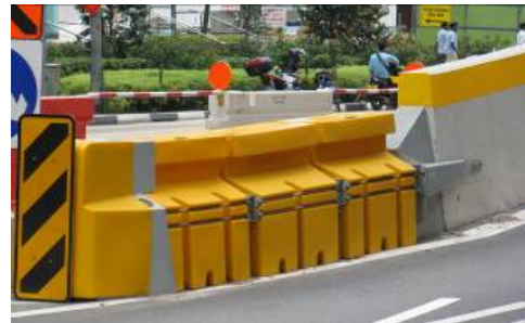
Use of crash cushion to shield the leading terminal of the concrete safety barrier
