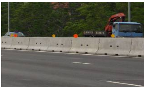
Example of pre-cast concrete safety barriers
