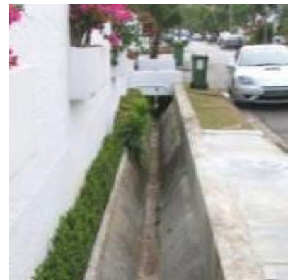
ABOVE: Open Composite channel drain beside footpath
