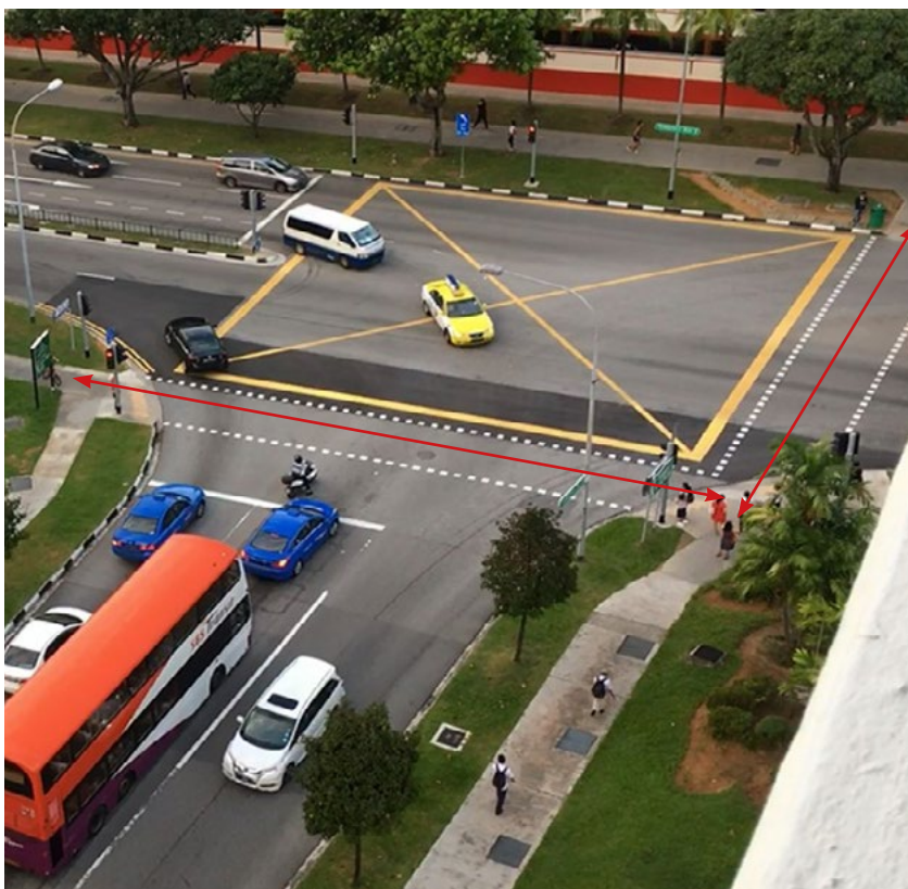
LEFT: Example of a limited crossing leg at a T-junction due to traffic and safety considerations.
