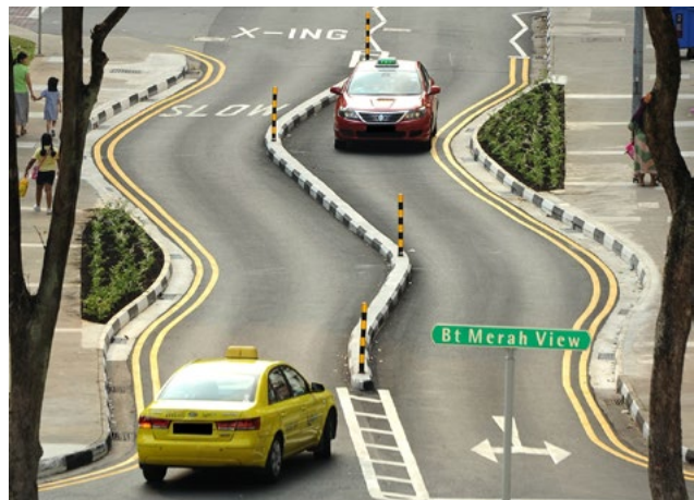
After: Chicane at Bukit Merah View
