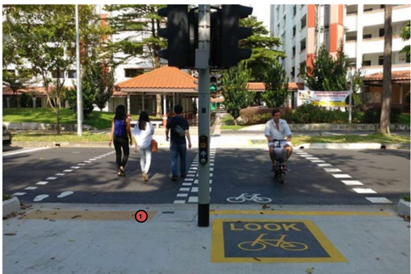
ABOVE: Placement of tactile tiles at crossing
