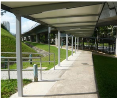
ABOVE: Cantilevered roof with column sited nearer to developments
