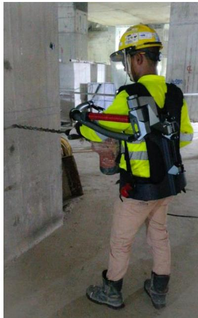
Fig. 2 Exoskeleton to help redistribute the weight of heavy equipment carried by workers
