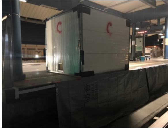
Figure 27: Localised noise enclosure erected for drilling works on existing LRT station
