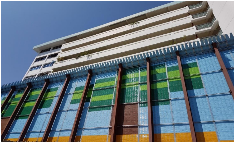
Figure 20: Flat Wedged Noise Barrier installed to mitigate noise.
