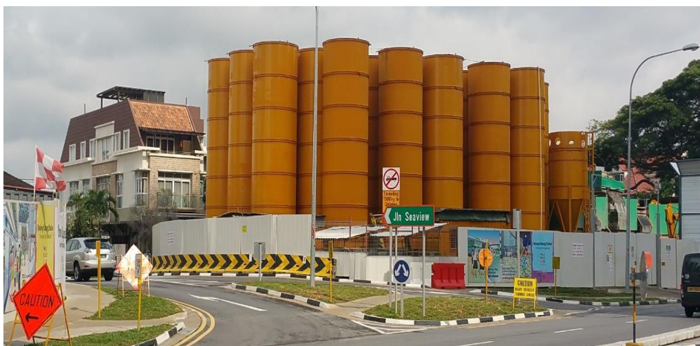
Figure 13: Silos was positioned to act as noise mitigation barrier.
