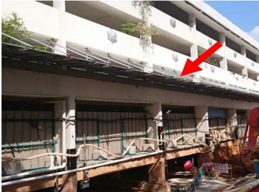
Figure 22: Noise panels was used to construct roof canopy along the corridor
