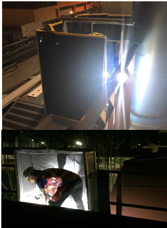
Figure 28: Portable noise barrier in place for works on existing MRT viaduct (bottom)
