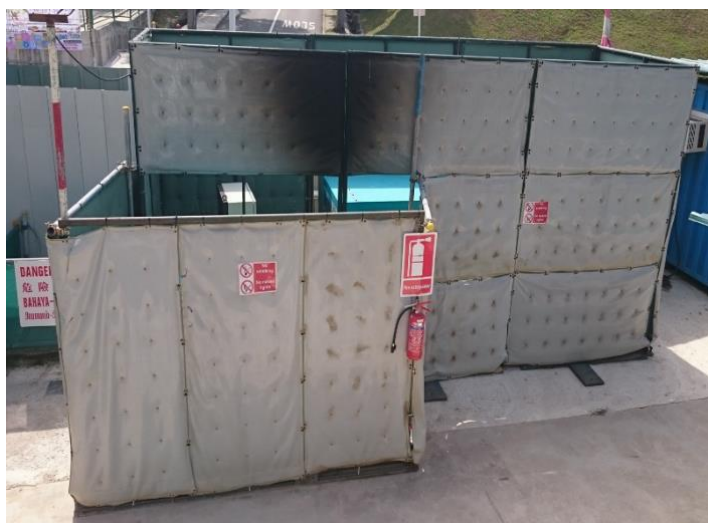
Figure 26: Noise blanket with acoustic foam erected to reduce noise from generator
