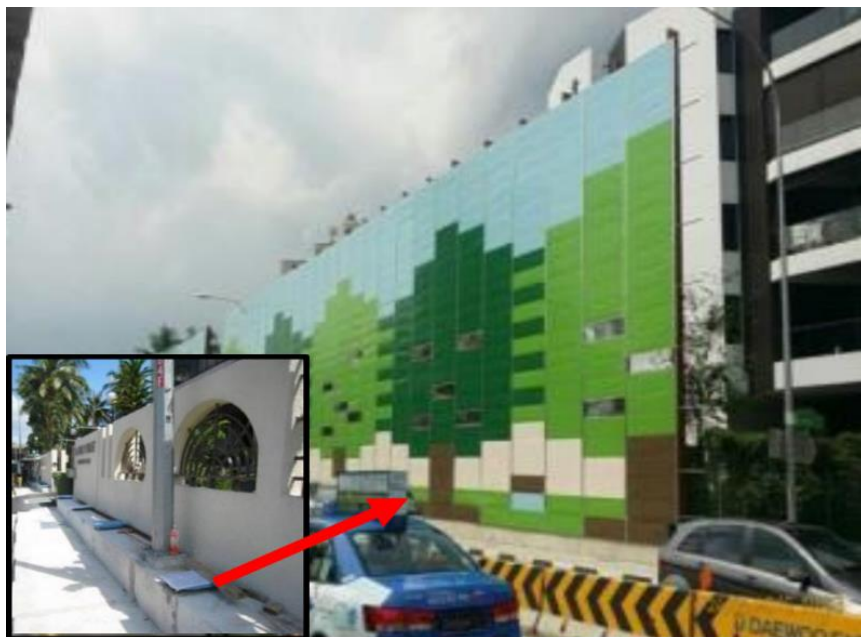
Figure 23: Noise barrier constructed with a narrow strip footing to overcome space constraint
