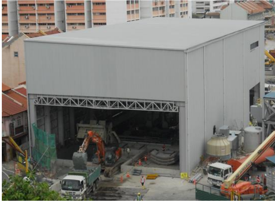
Figure 18: Full noise enclosure with rolling shutter installed at launch shafts for noisy tunnelling works
