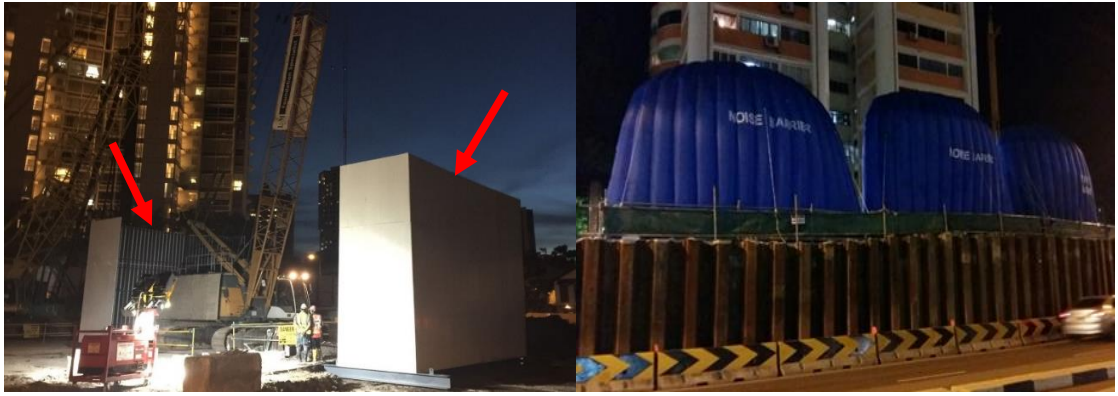
Figure 24: Portable and inflatable noise barriers are in place for localised works.
