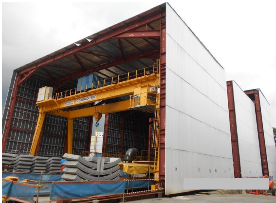
Figure 19: Retractable noise enclosure installed at launch shafts for noisy tunnelling works
