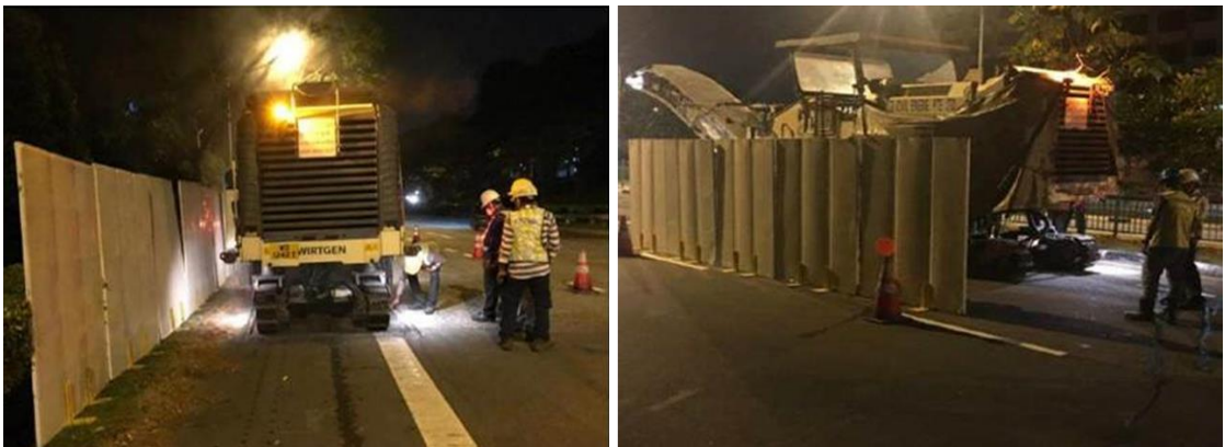
Figure 25: Portable noise barriers erected for localised road works
