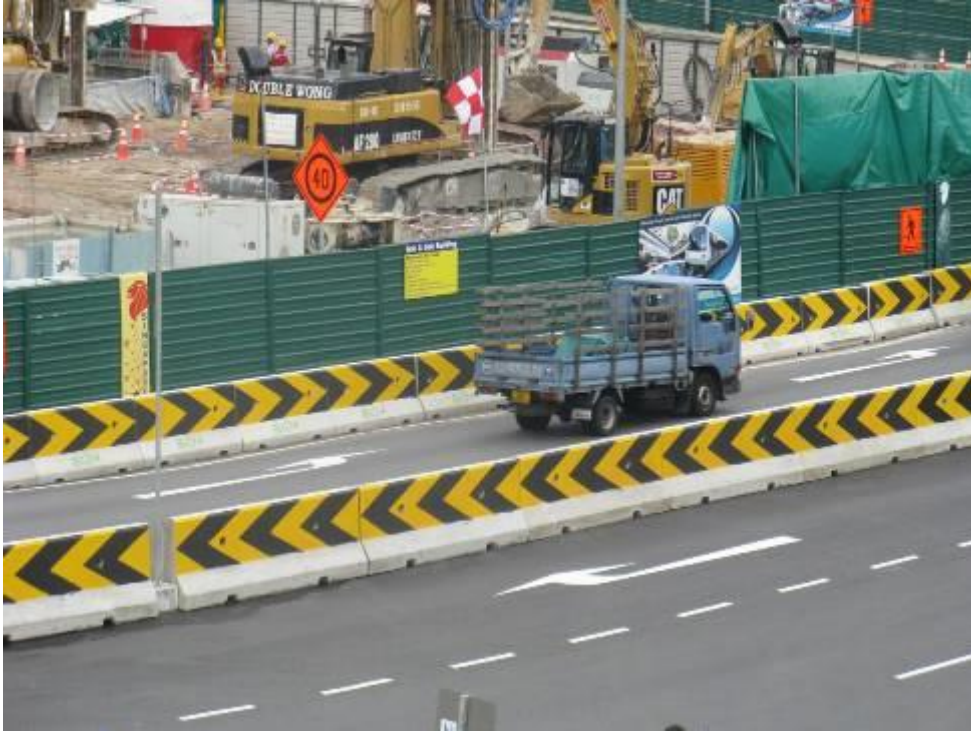
Concrete barriers use to protect workers against the possibility of vehicles crashing into site boundary
