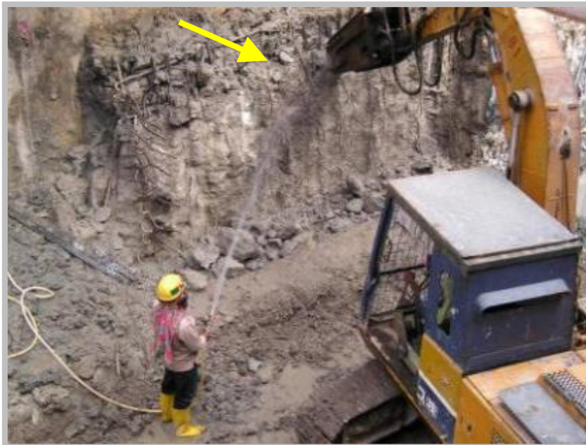
Arresting of dust at source using recycled water
