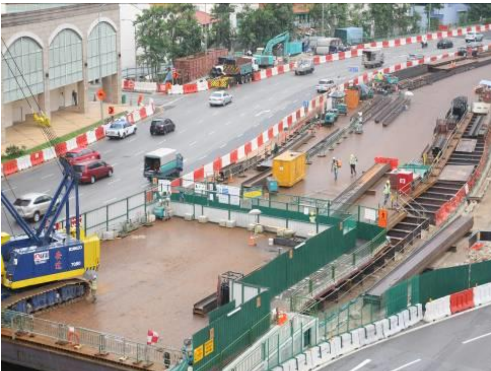
Good housekeeping around worksite
