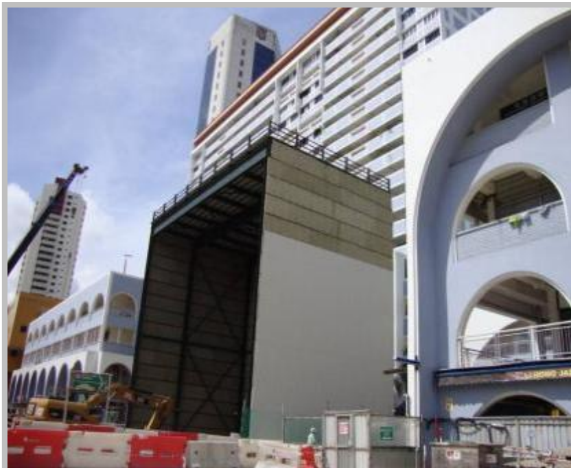
Large acoustic enclosures used for noisy activities / machineries (For e.g. excavation activities, launch shaft) conducted near noise sensitive receivers)
