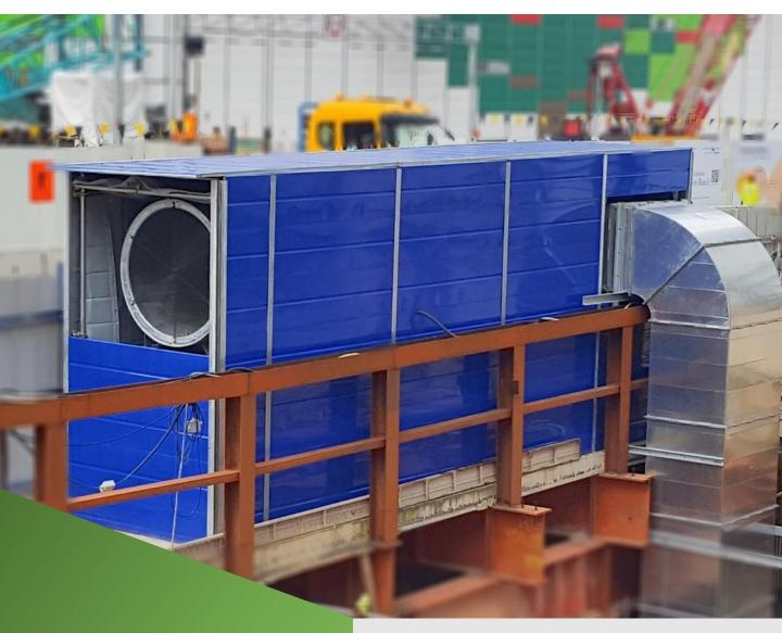
Noise Enclosure for Ventilation Fan Provide noise enclosure for ventilation fan
