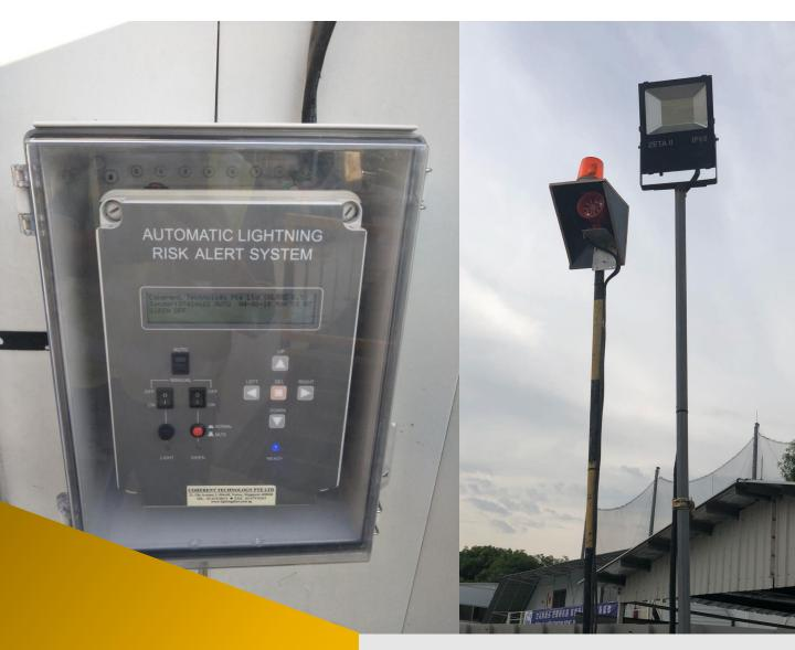
Automatic Lightning Warning System Provide real time lightning warning alert
