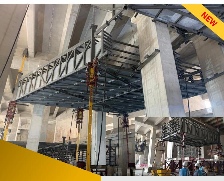
Hydraulic Jacking System Provide hydraulic jacking system for heavy modules.
