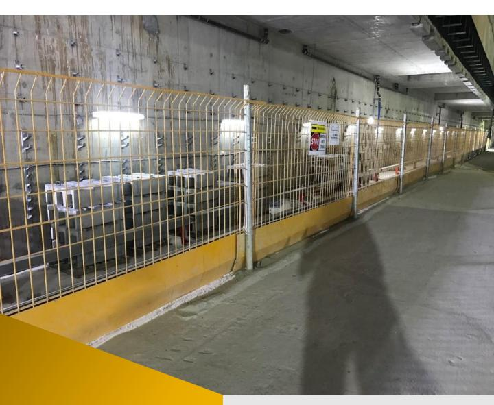
Proprietary Fall Protection System Provide fall prevention barricades
