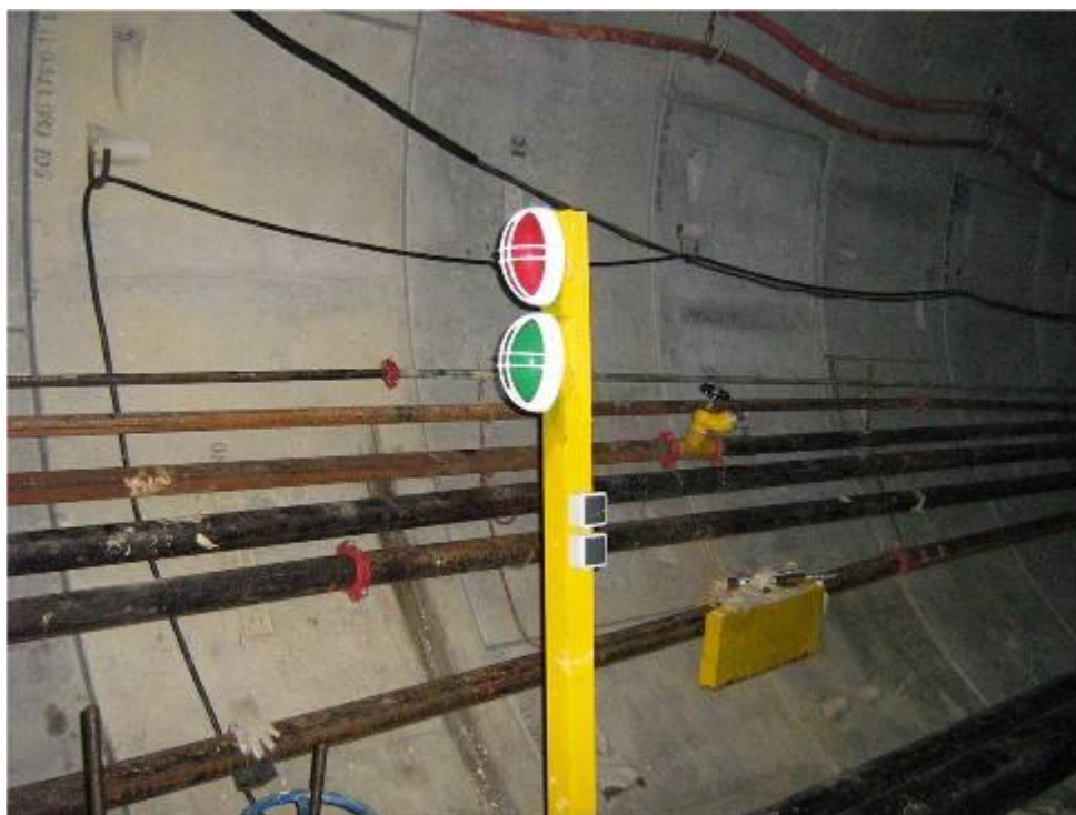
Red and Green signal light to regulate locomotive movement in the tunnel
