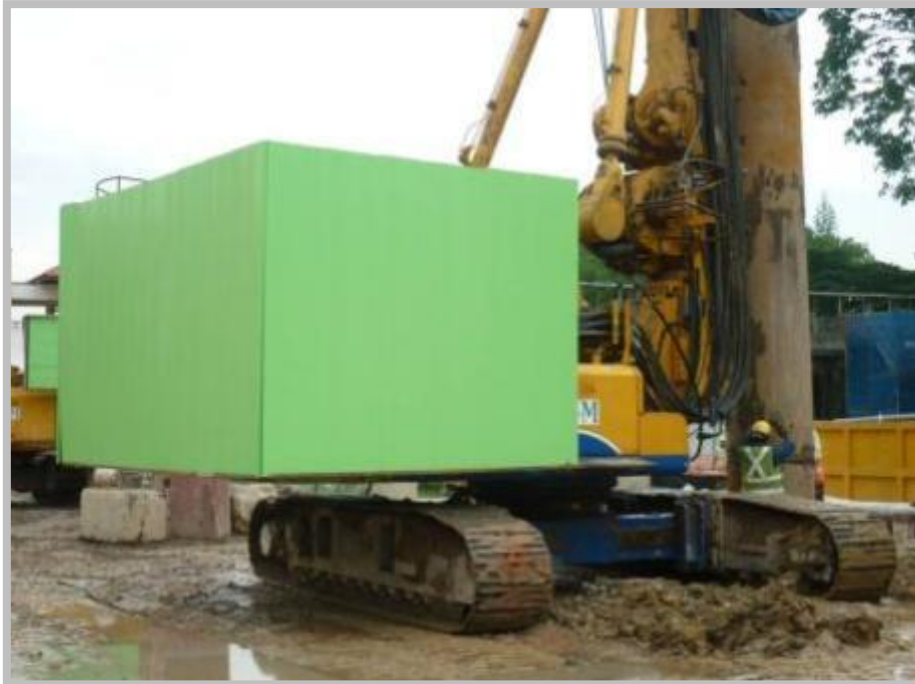
Noise enclosure on boring rigs
