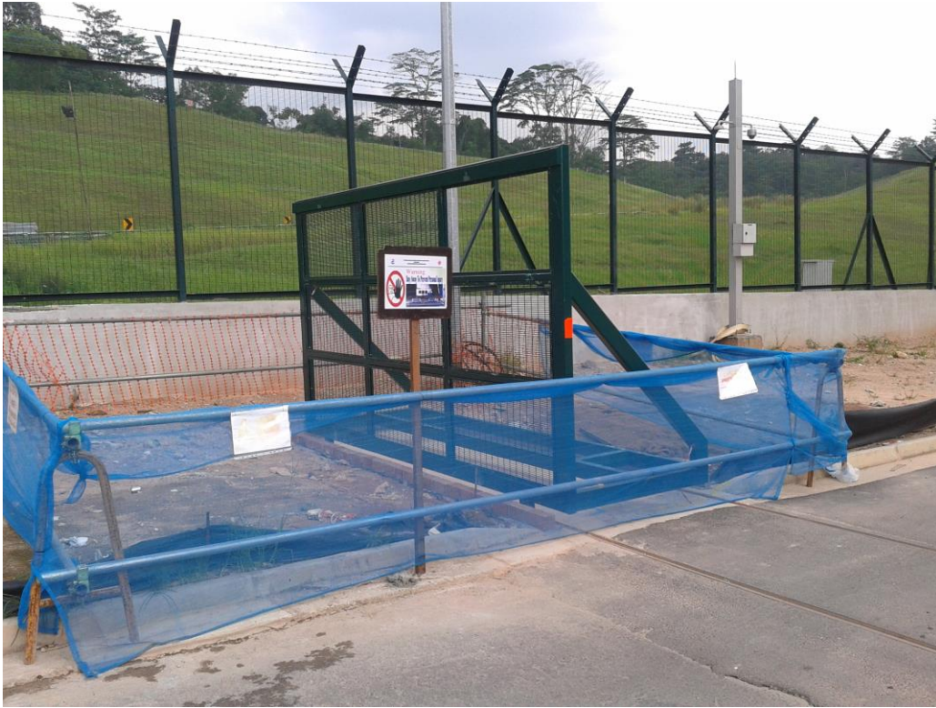
Cordon off work zone around gate installation
