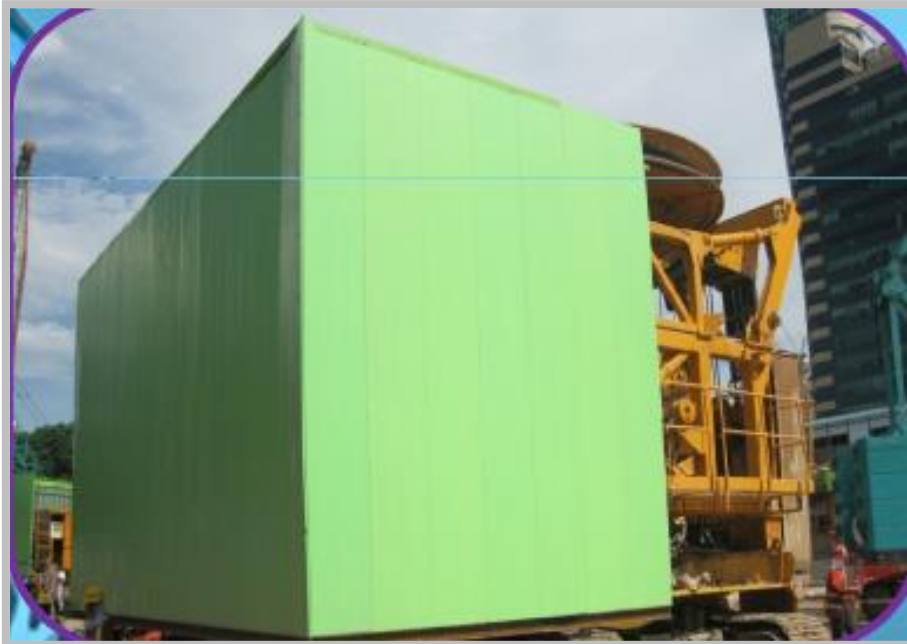
Noise enclosure on D-wall cutter machine
