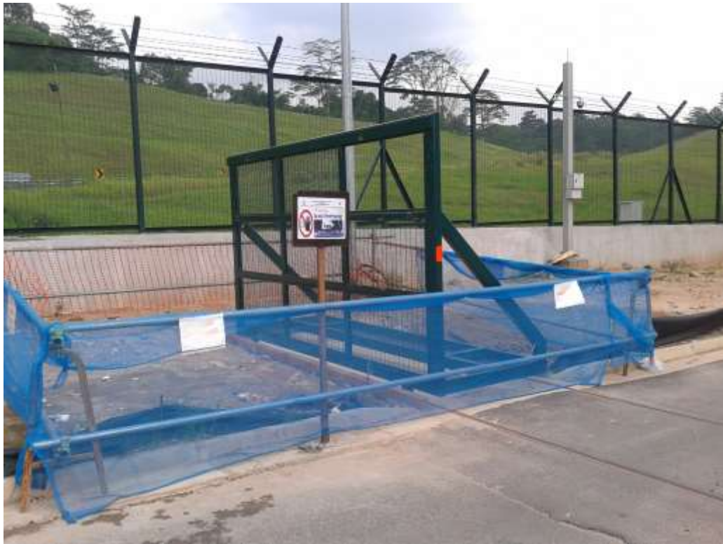
Cordon off work zone around gate installation
