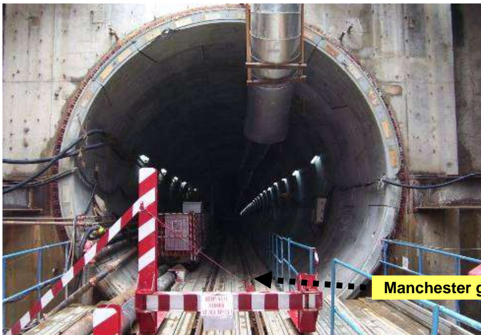
Manchester gate installed to regulate movement of locomotive in tunnel
