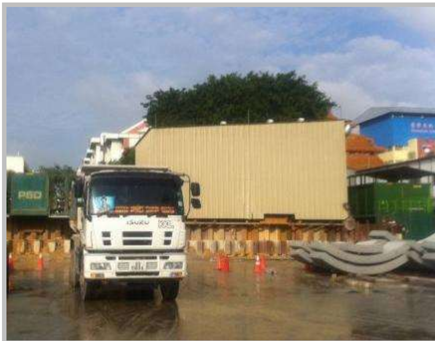
Large acoustic enclosures on slurry treatment plants
