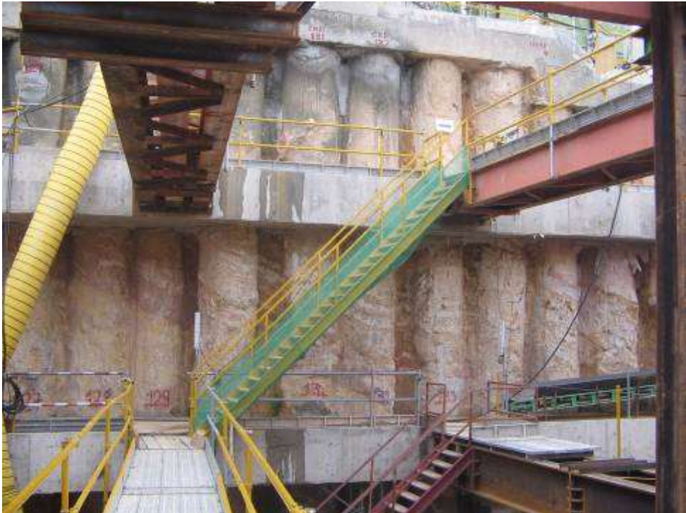
Steel staircase with unobstructed headroom and netting wrapped around handrail and underneath of steps to prevent loose material from falling through
