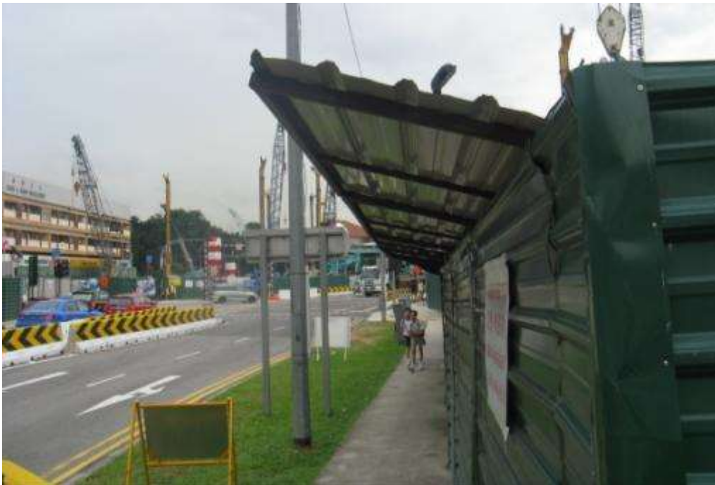
Overhead shelter provided when work is carried out near hoarding to protect the public from any falling objects
