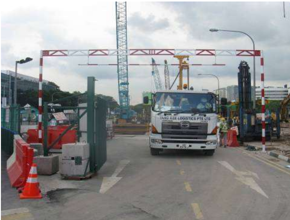
Height Limit Gantry installed at site entrance / exit to ensure the total height of the vehicle does not exceed 4.5m
