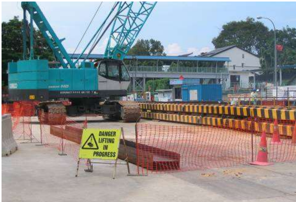
Lifting activity is cordoned off and warning signage is placed to warn personnel against entering the area
