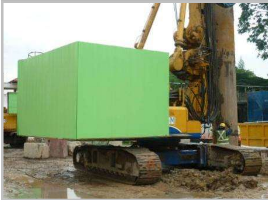
Noise enclosure on boring rigs
