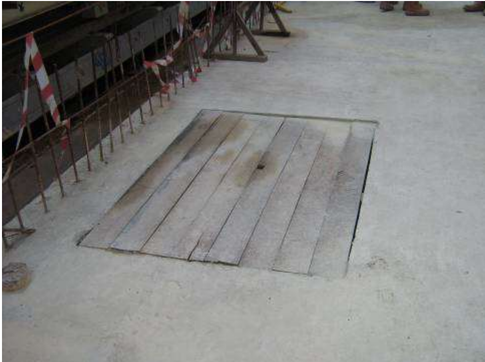
Floor opening cover is flushed and secured against moving
