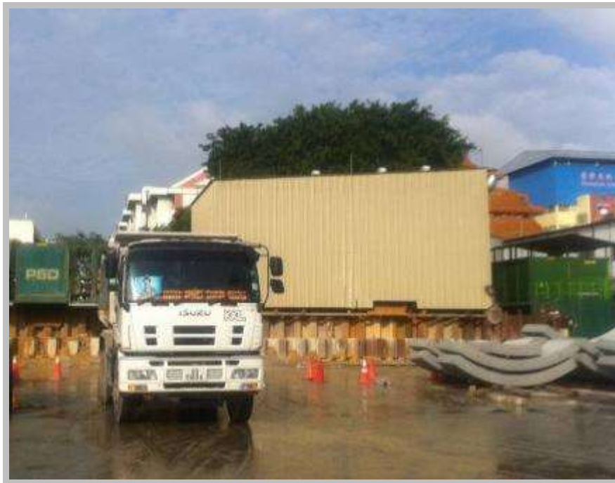
Large acoustic enclosures on slurry treatment plants
