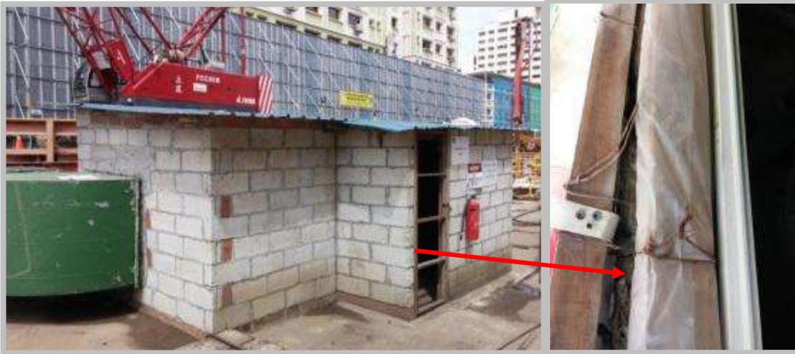
Use of celcon block walls with built-in rockwool to house noisy ventilation fan
