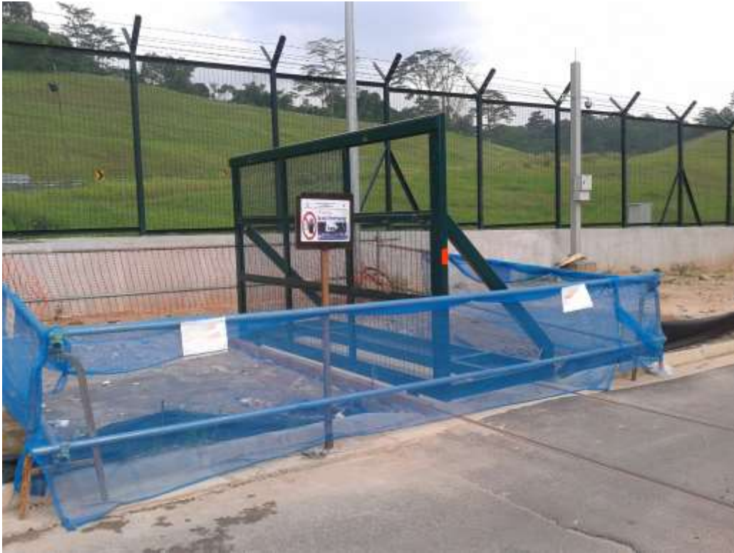
Cordon off work zone around gate installation
