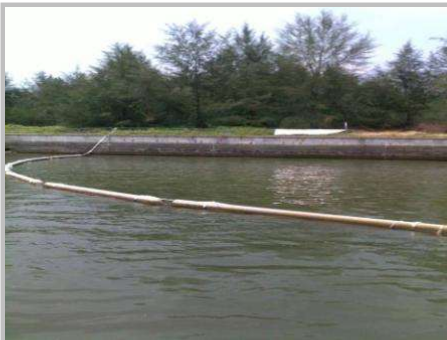
Adequate use of turbidity curtain for works near water-bodies / waterways
