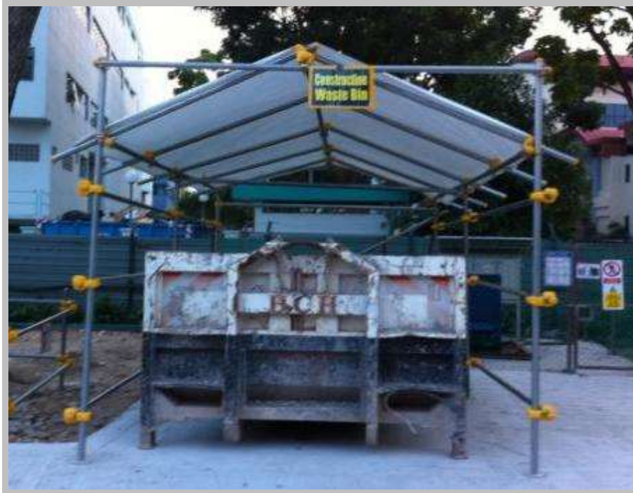
Provision of adequate and sheltered bins for containment of wastes
