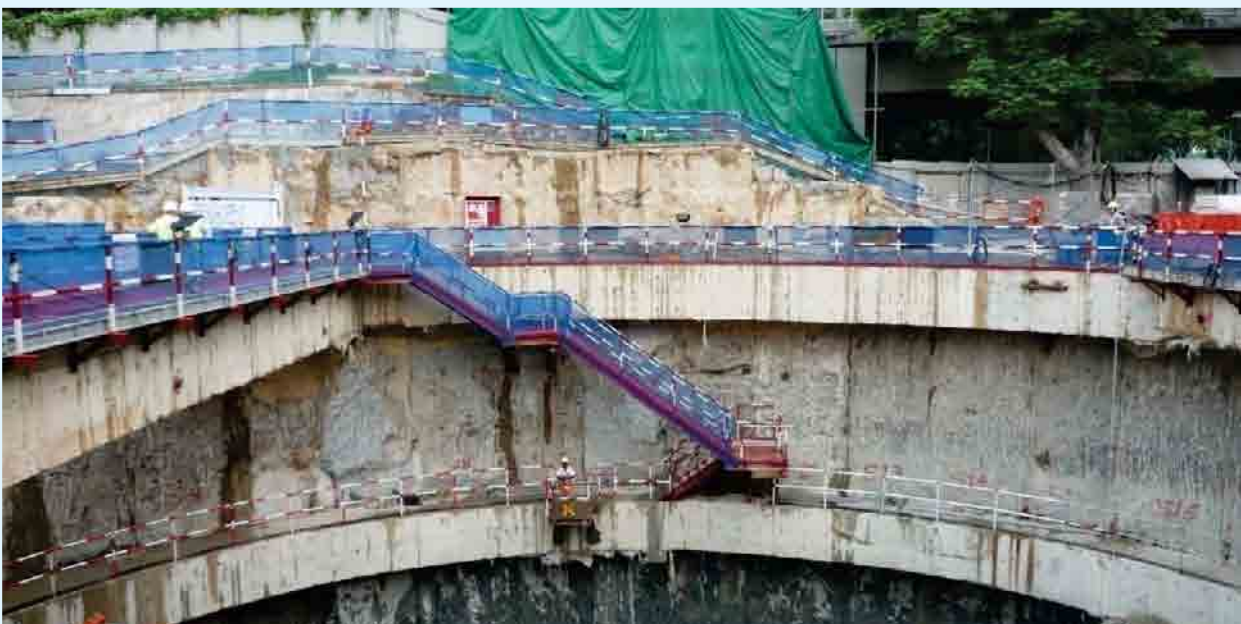
Notices and guardrail provided at excavation zone
