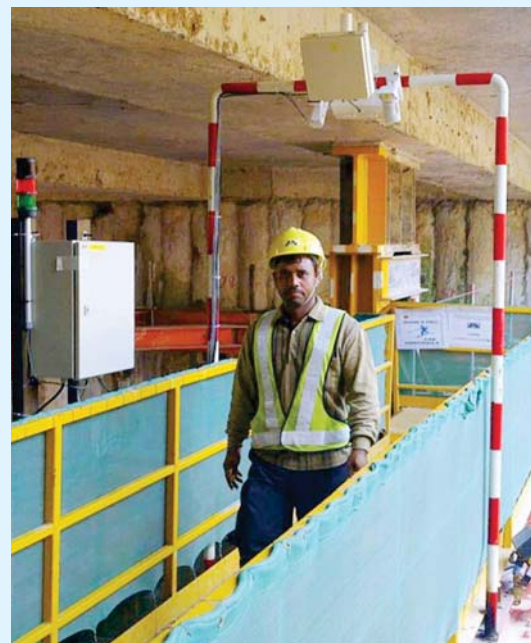
RFID gantry was erected to track access to and egress from confined space
