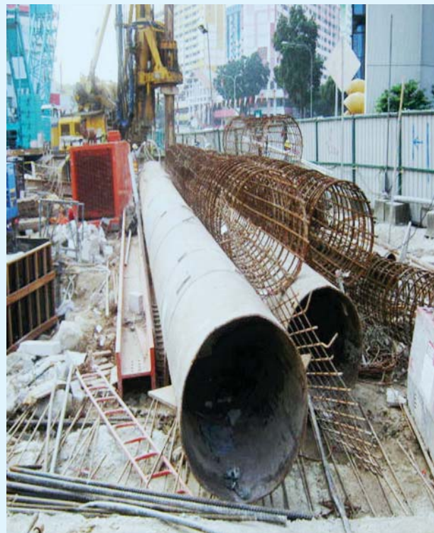
Improper storing and stacking of unused materials
