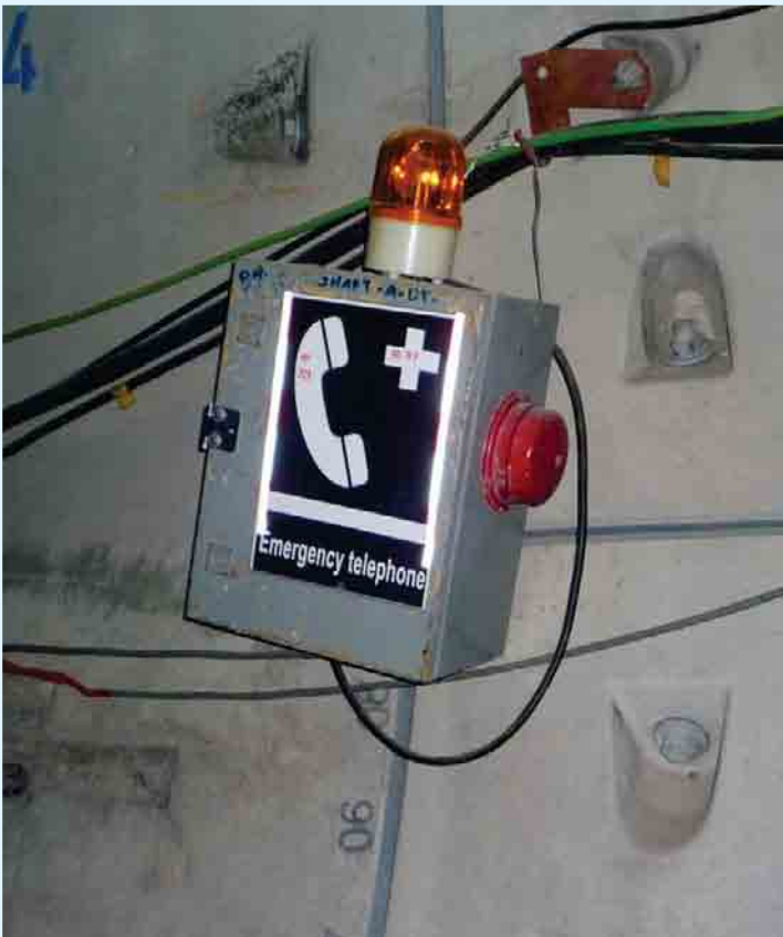
Emergency telephone provided in tunnel
