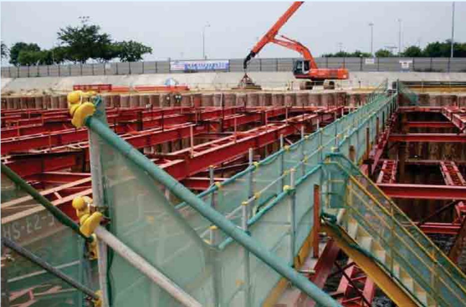
Proper walkways provided along struts
