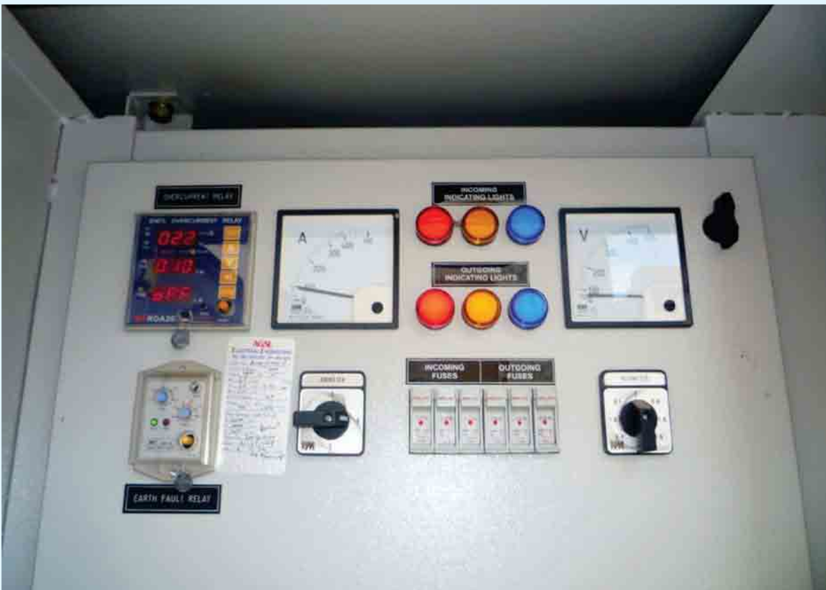
Distribution board with Residual Current Circuit Breaker (RCCB) and other safety devices
