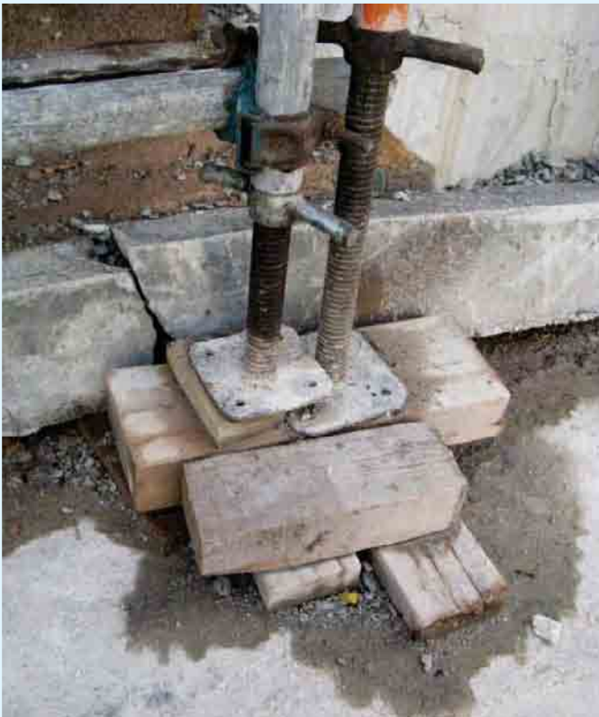
Stacked timber pieces as foundation is not acceptable
