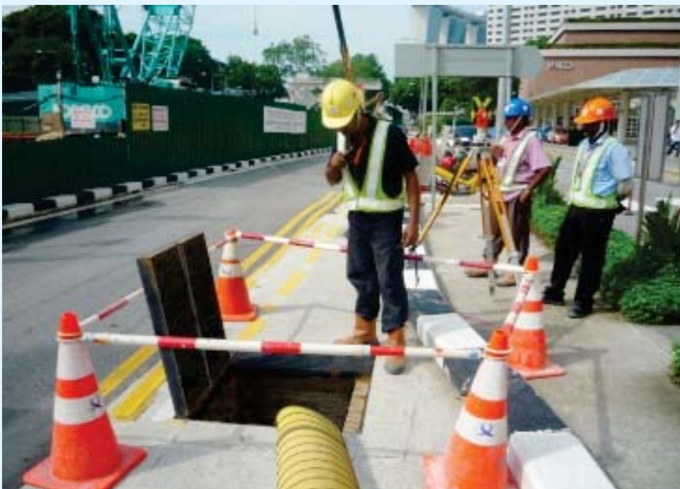
Confined space attendant maintaining regular contact with worker inside confined space
