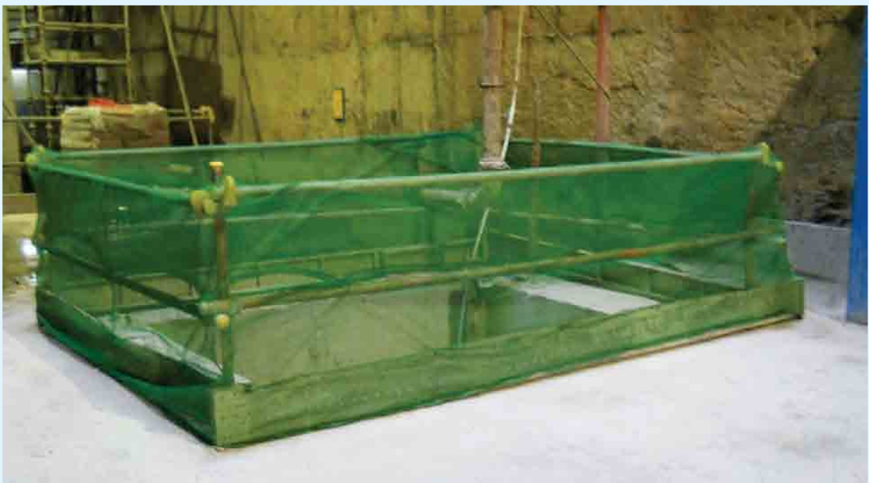
Provision of standard method of railings, toeboards and netting. Height of railings to be at least 1.1m high
