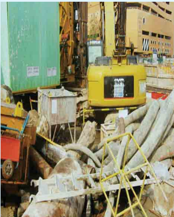
Improper storing and stacking of unused materials
