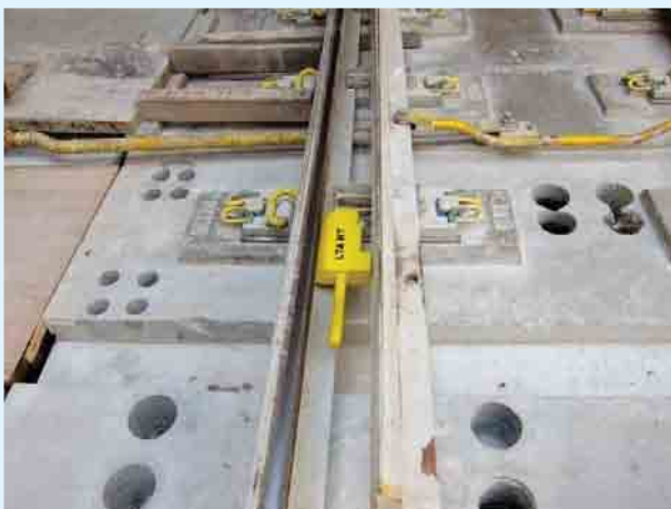
Point secured with G Clamp & Point Scotch for a Safe Shunting movement
