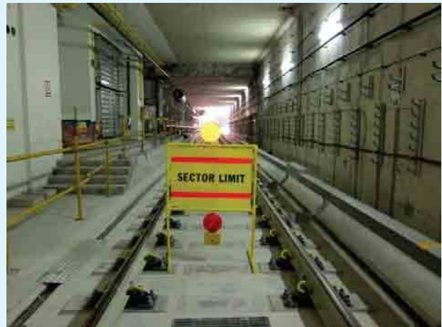
Sector Limit Board with flashing light is used by the Possession Master who has full control of a sector for demarcation purposes
