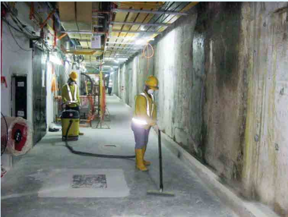
Using vacuum cleaner to prevent dust accumulation in the station box
