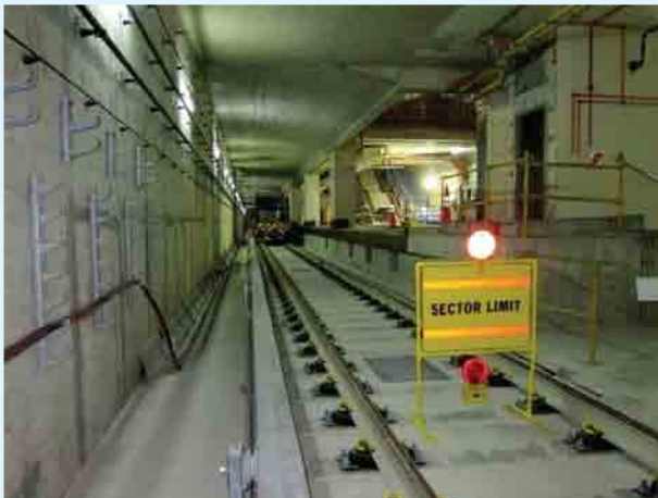
Sector Limit Board with flashing light is used by the Possession Master who has full control of a sector for demarcation purposes
