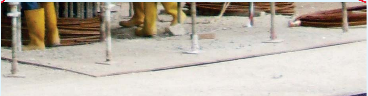
Scaffold erected on a proper foundation
