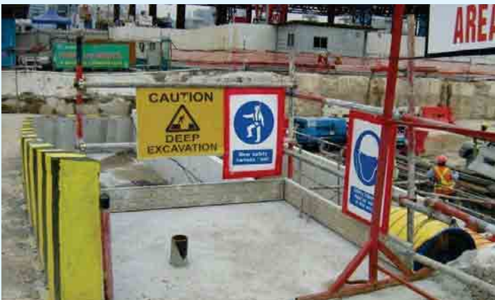
Notices and guardrail provided at excavation zone
