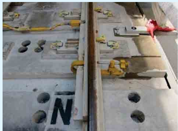
Point secured with G Clamp & Point Scotch for a Safe Shunting movement
