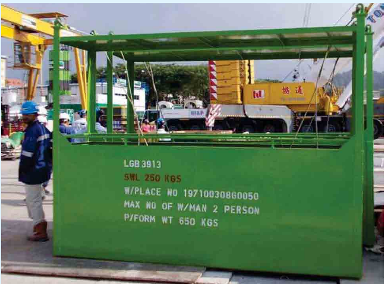
Example of man-riding cage which is capable of taking a stretcher and two persons together
