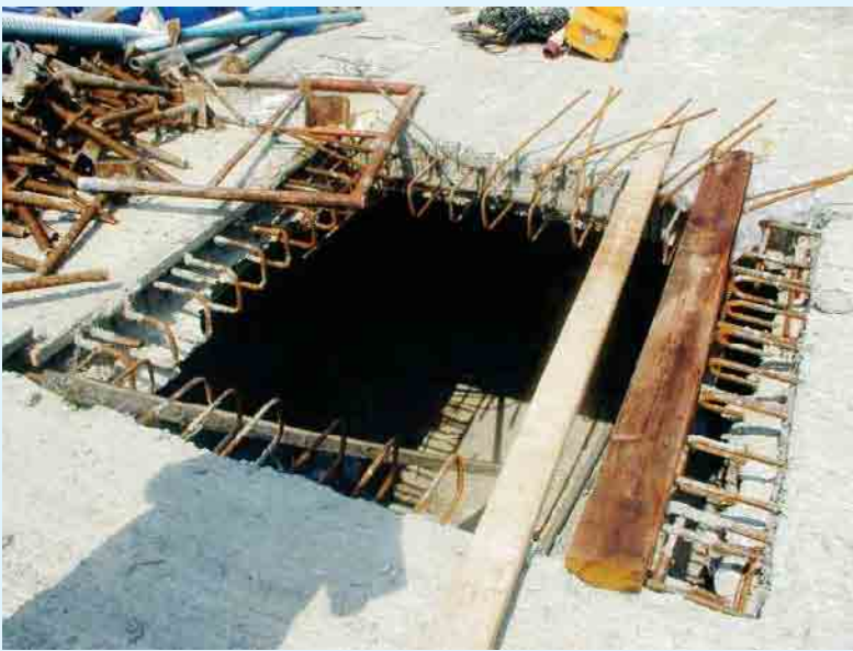
Opening in floor is not covered to prevent fall
