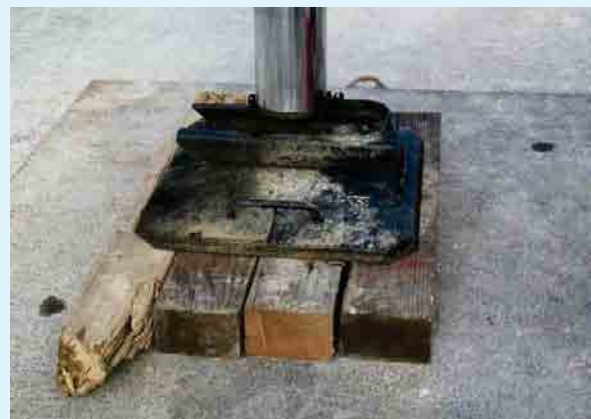
Outriggers resting on plank
