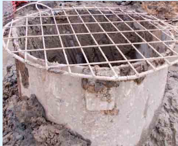
Opening in floor is not covered to prevent fall
