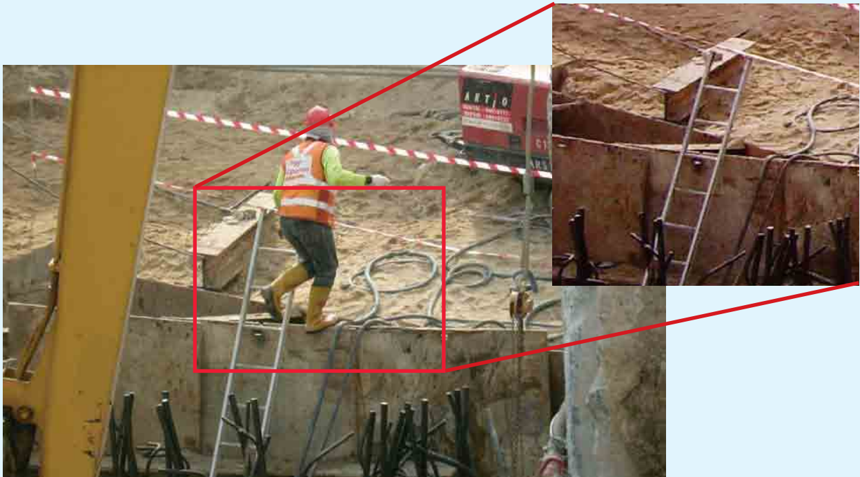
No proper landing platform, ladder not secured
