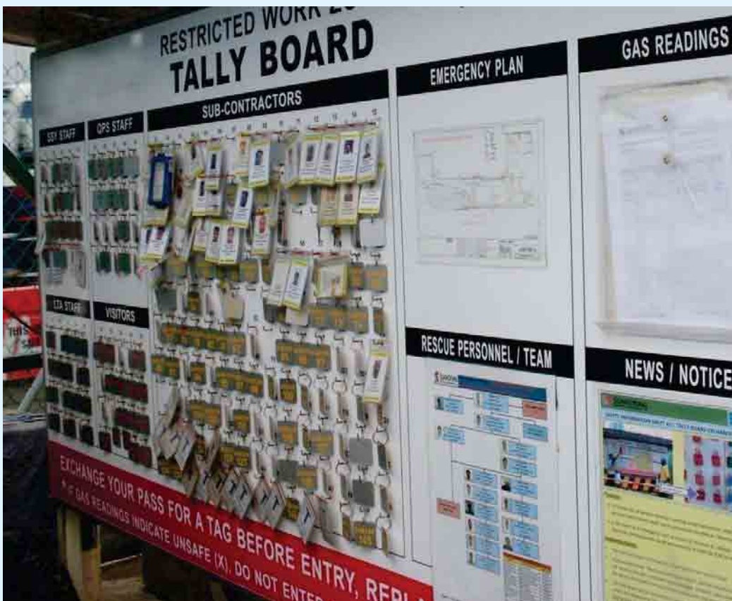
Tally board placed near excavation opening
