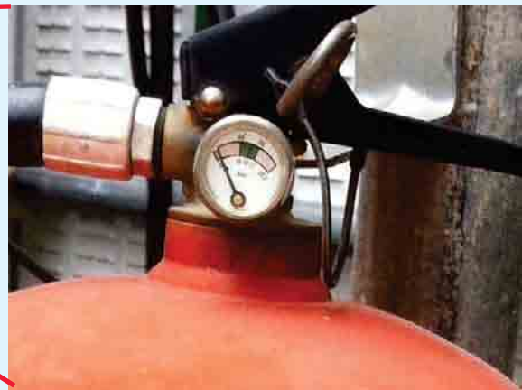
Fire extinguisher was not maintained
