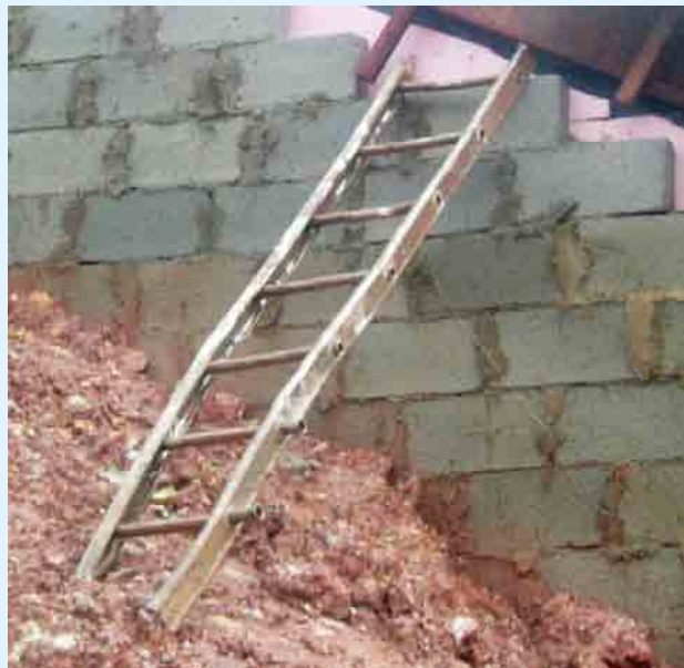
Crooked and unsecured ladder should be removed from site
