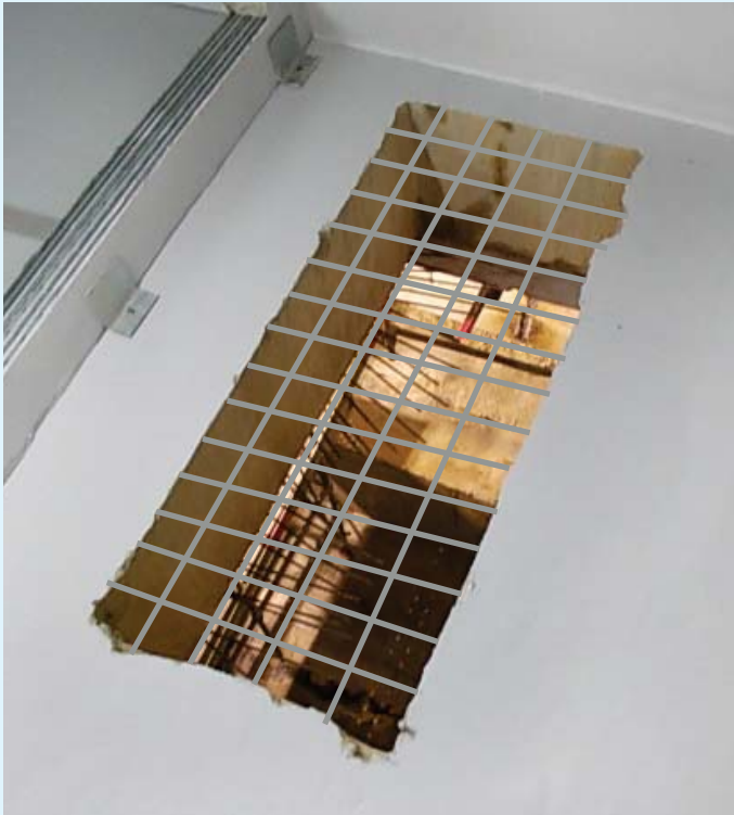
A13 mesh, fixed to the top steel and cast into the slab
