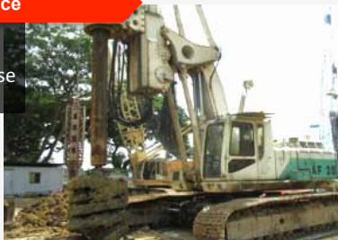
Bored piling works
