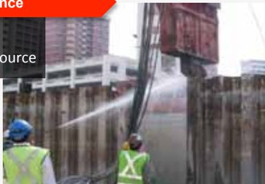
Installation/Extraction of sheet piles
