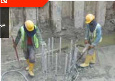
Mechanical hacking works
