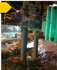
Deep cement mixing works
