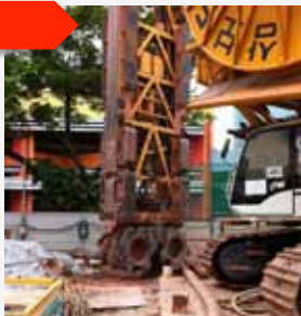
Diaphragm wall works
