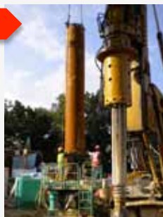
Installation/Extraction of casings
