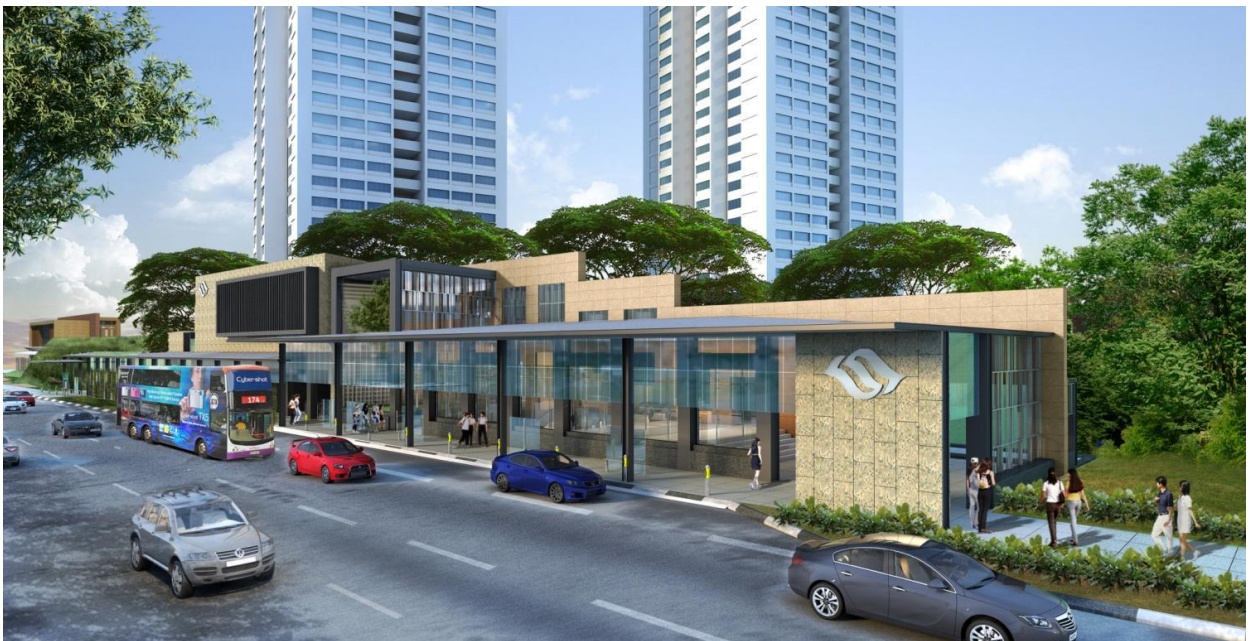
Entrance of Havelock Station
