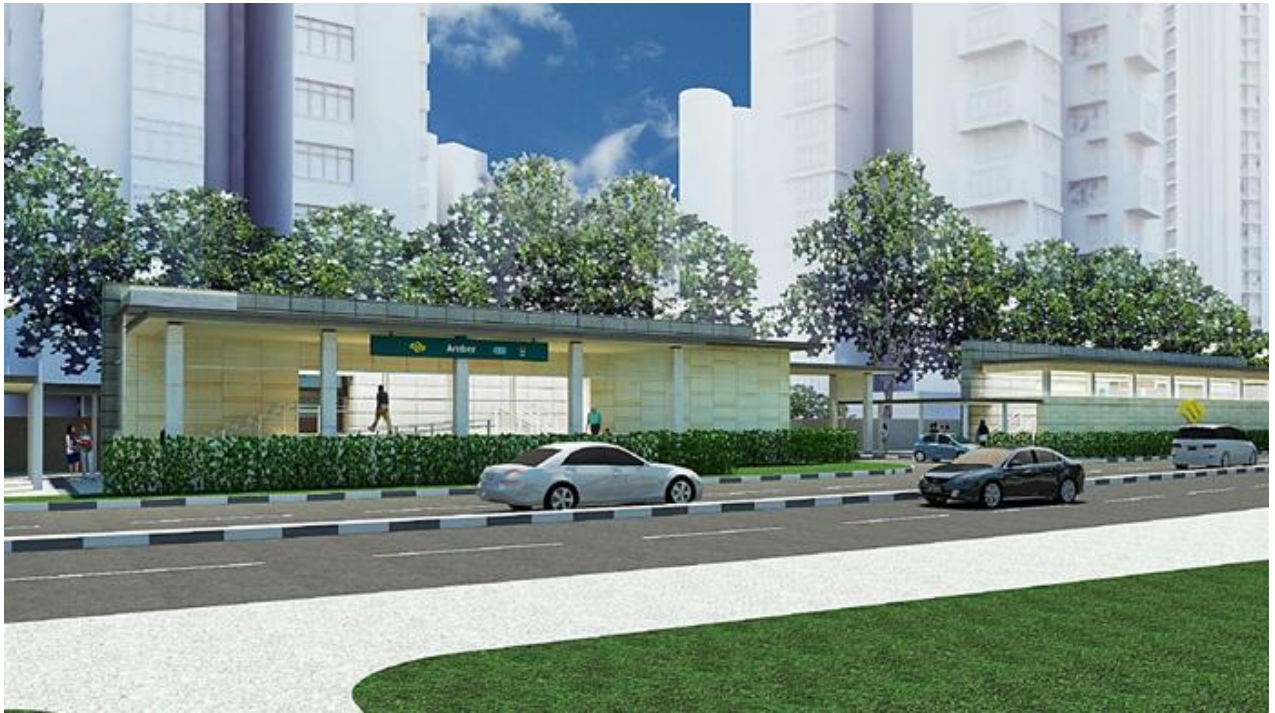
Entrance of Amber Station
