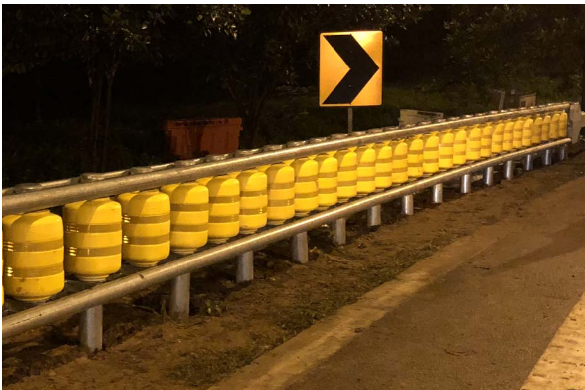
Roller Barrier System along a stretch of the slip road between PIE(Tuas) and BKE(Woodlands)
