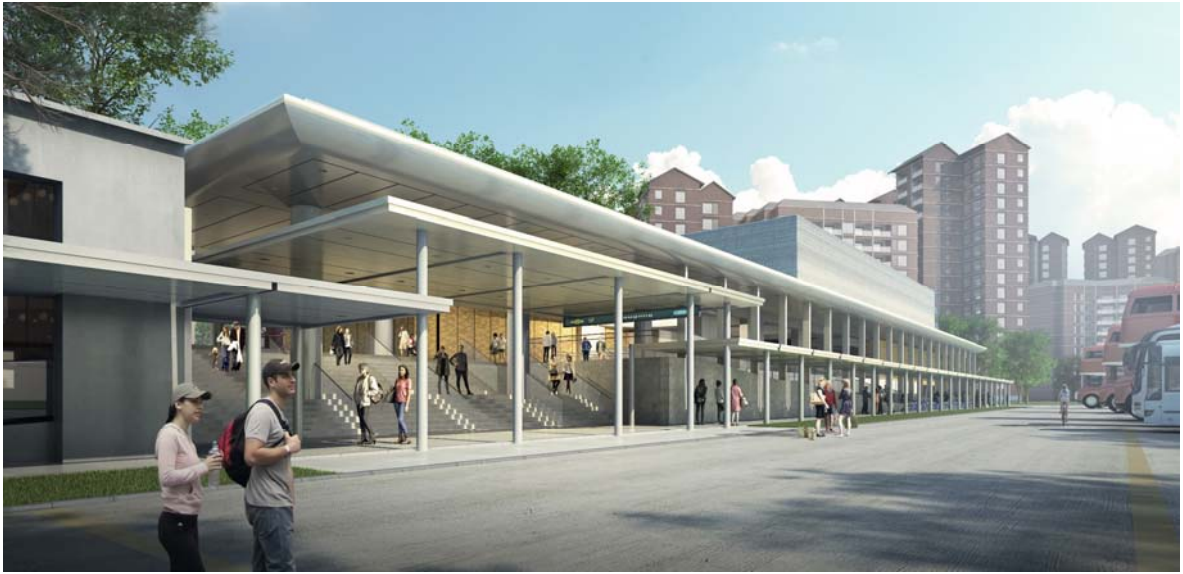
CRL Hougang station entrance
