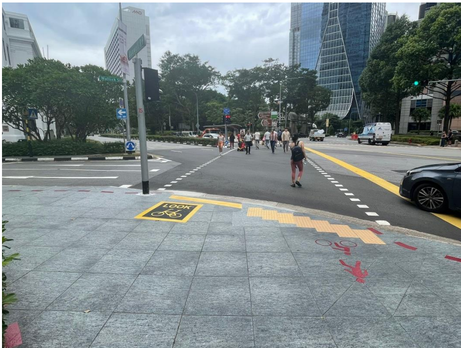
Signalised crossing at Wallich St/ Maxwell Rd – after widening
