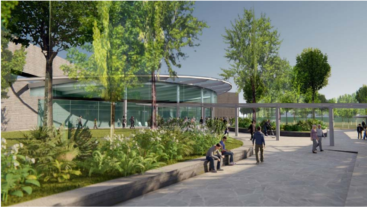
CRL-Aviation Park station
