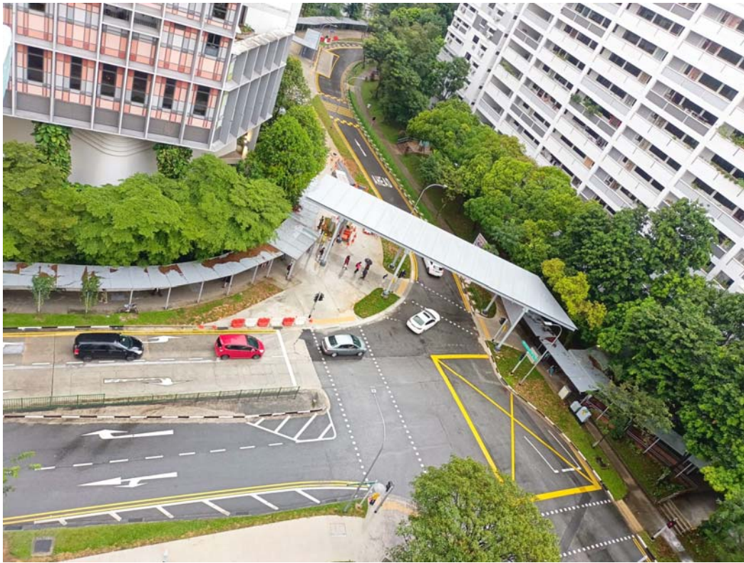
After: Works to partially pedestrianise Woodlands Ring Road are almost complete, with covered linkways, wider footpaths and a new bus stop
