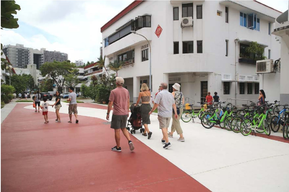
After: Civil works to partially pedestrianise Eng Hoon Street are completed, with planting and installation of street furniture to follow
