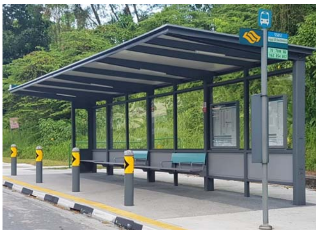
Completed bus stop at Yio Chu Kang Road
