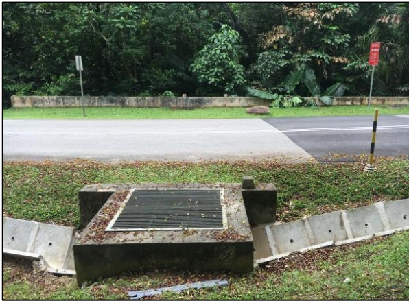
Inlet connecting roadside drains and Stream Ma
