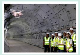
Using drones for tunnel inspections
