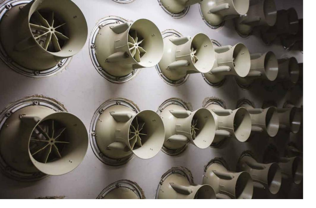
For each of the 15 DTL stations that are also Civil Defence public shelters, including the Tampines East station pictured here, an overpressure regime and airflow test was conducted. Picture: LTA
