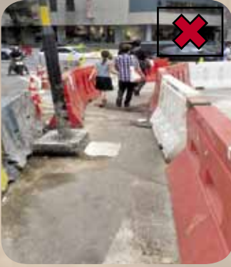
Figure 3: Obstruction along the pedestrian footpath
