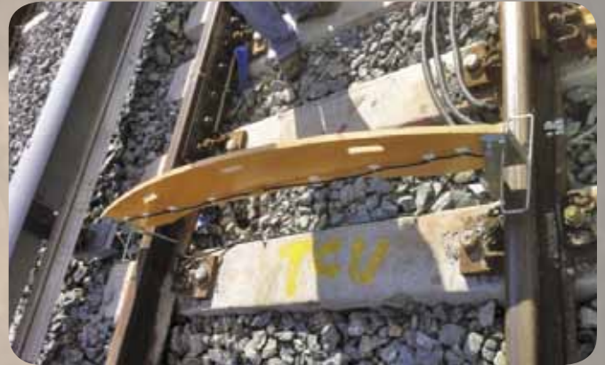
Figure 4: Track Circuit Shunt Test
