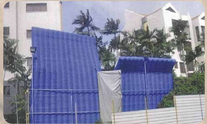
Figure 2: Contract 923 Samsung C&T Corporation "Inflatable Noise Barriers"
