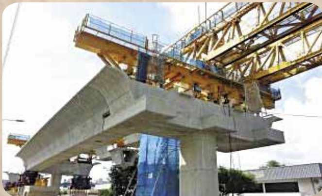
Figure 5: LG at Joo Koon Circle with beam launched
