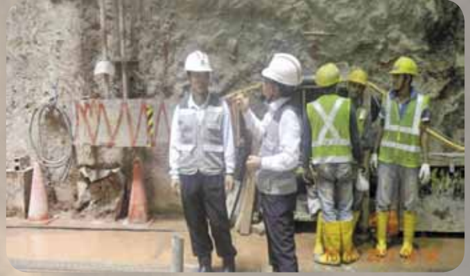
Figure 7: Project Director safety walks
