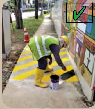
Figure 4: Ramp or uneven surface painted with luminary colour to alert the pedestrian
