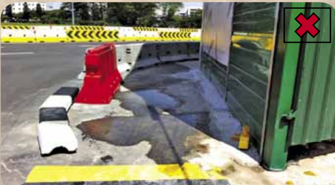
Figure 6a: Water ponding due to uneven surface
