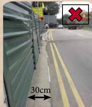
Figure 7a: Insufficient width of footpath
