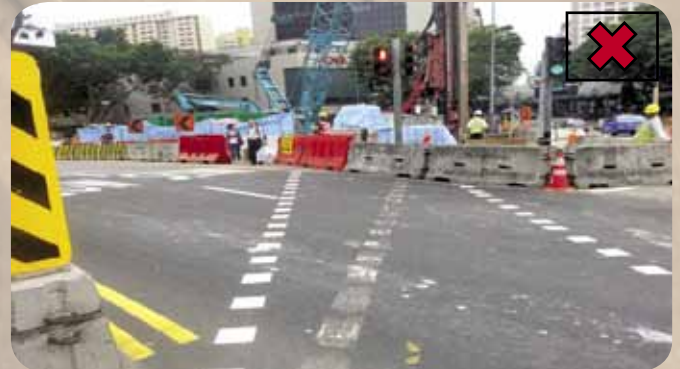
Figure 2a: Misaligned pedestrian crossing path with waiting area
