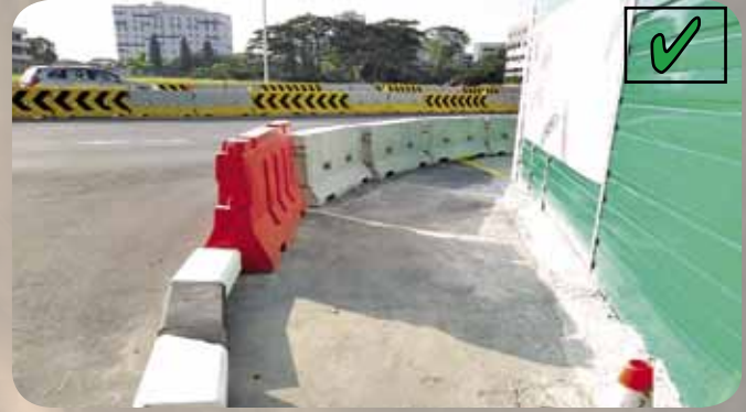
Figure 6b: The surface of walkway is graded to prevent water ponding
