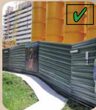
Figure 5b: Lighting facility provided at night along the footpath
