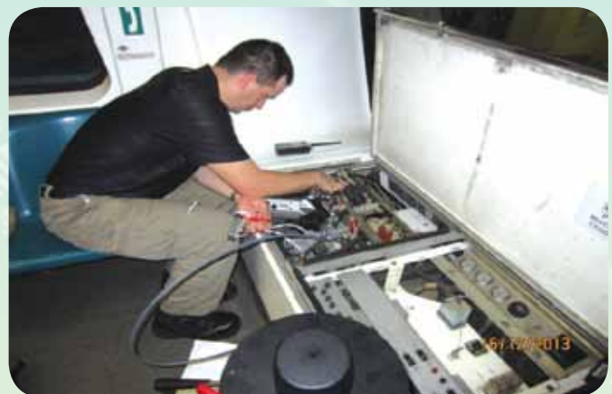
Figure 2: Testing the newly retrofitted kit and antenna during Stage 2 Radio Migration
