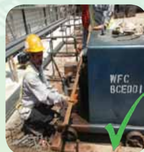
Figure 1: Wear suitable gloves when handling rebars
