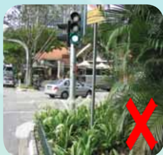
Figure 5a: The overgrown shrubs at the roadside verge of the junction is obstructing the motorists' visibility of the pedestrians crossing this junction
