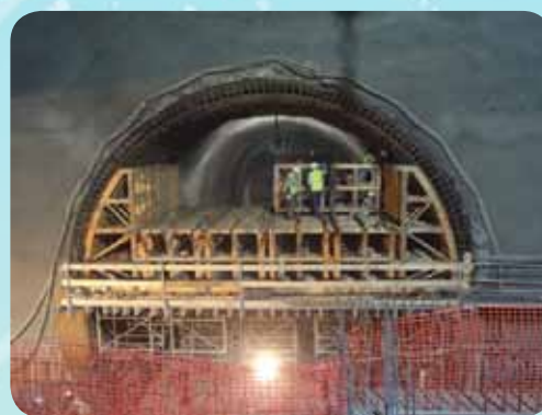
Figure 5: Conventional timber formwork system used for the construction of the permanent lining of a mined tunnel
