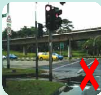
Figure 8a: Waterponding occurs due to inadequate drainage at the traffic island
