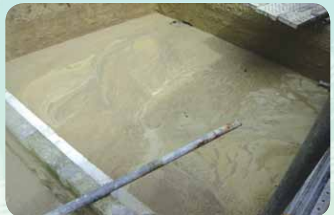
Figure 4: Tunnelling wastewater was channelled to holding pond leading to ECM treatment plant
