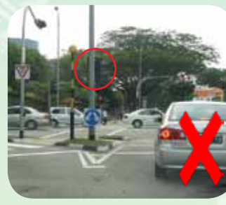
Figure 3a: Traffic signal pole is obstructed by street lighting pole that is located on the same traffic island
