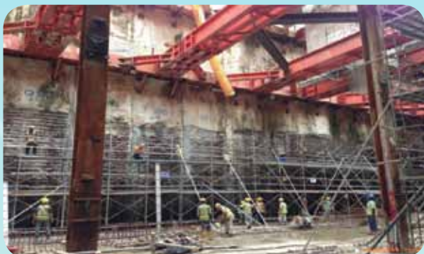
Figure 3: Conventional method of using scaffold and pneumatic breakers
