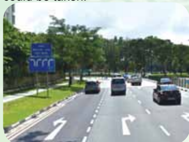
Figure 6: Motorists are informed of the exclusive turning lanes and adequately guided at a junction by providing a lane indication sign
