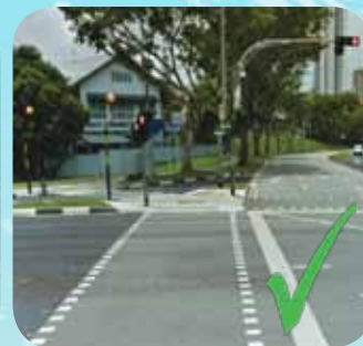
Figure 7b: The pedestrian crossing lines are painted within the traffic island, thus preventing pedestrians from waiting outside the island
