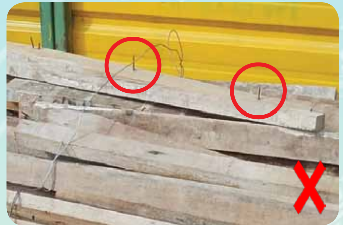
Figure 8: All exposed nails should be removed / made safe
