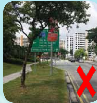
Figure 2a: Directional sign is obstructed by tree and street lighting pole
