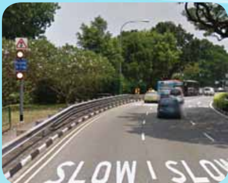
Figure 4: Providing Advance Warning Light along a bend helps to forewarn motorists of the changes in traffic signals in the junction ahead
