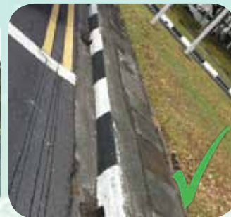
Figure 8b: Drainage inlets have been provided along the edge of the traffic island to channel away surface runoff adequately
