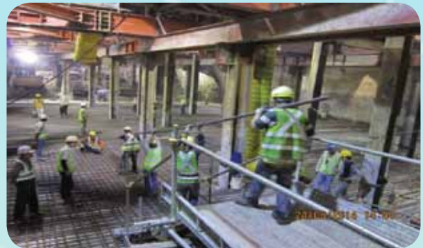
Figure 1: Conventional way of fixing rebars for ground slab
