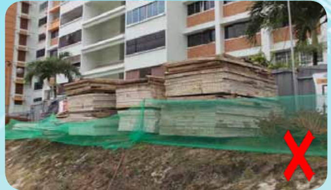
Figure 7: Do not stack materials at the edge to prevent tipping
