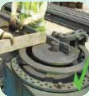
Figure 5: Use timber planks to wedge rebars
