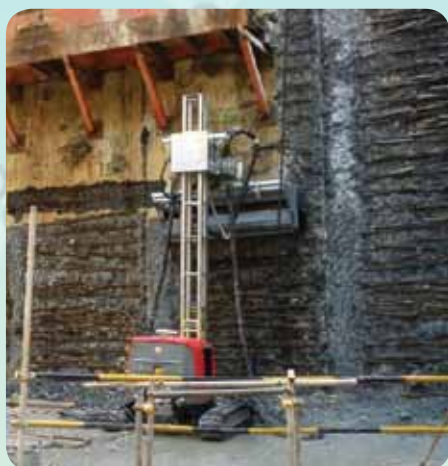
Figure 4: Use of high pressured water jet to remove concrete layer to expose rebars for integration with skin wall, slab and beam
