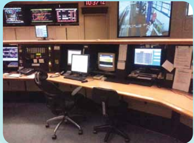
Figure 1: New ORS (Operational Radio System) PC installed during Stage 1 Radio Migration
