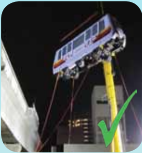
Figure 3: Tagline used to control of swing of load
