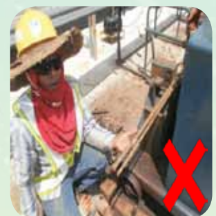
Figure 2: Do not use bare hands when handling steel or sharp materials
