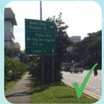
Figure 2b: Directional sign is unobstructed by trees or street furniture
