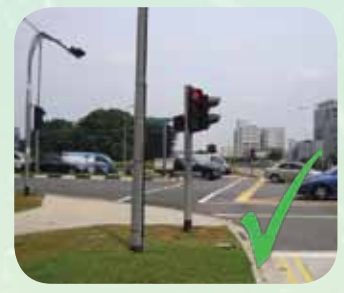
Figure 3b: Street lighting pole is located away from traffic signal pole to ensure unobstructed visibility of the traffic signal pole
