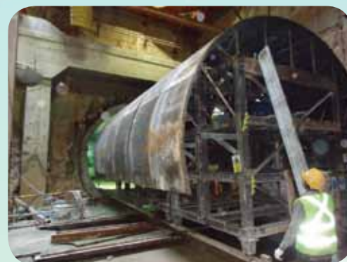
Figure 6: A Self Propelled Hydraulic Formwork System
