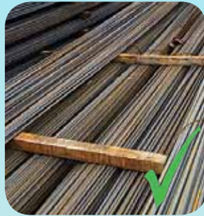
Figure 4: Timber spacers between stacked rebar for easy rigging
