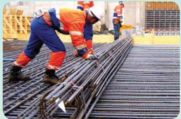
Figure 2: Workers rolling out a bundle of the 'rebar carpet'
