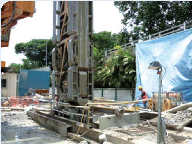
Figure 3: Diaphragm wall installation beside flyover
