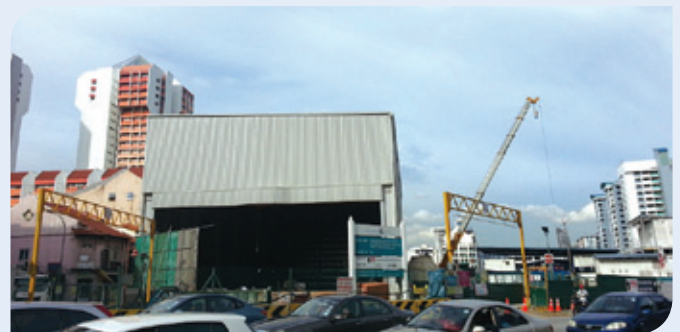
Figure 3: Launch Shaft Noise Enclosure
