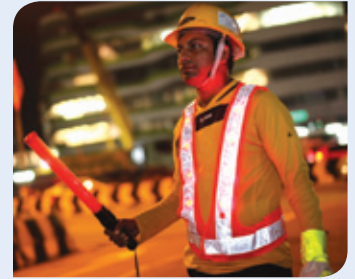
Figure 7: Traffic controller directing traffic at the construction site
