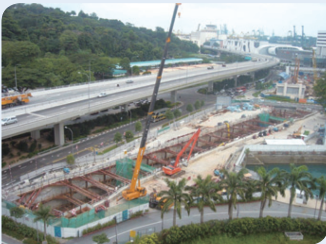
Figure 1: Excavation works beside flyover
