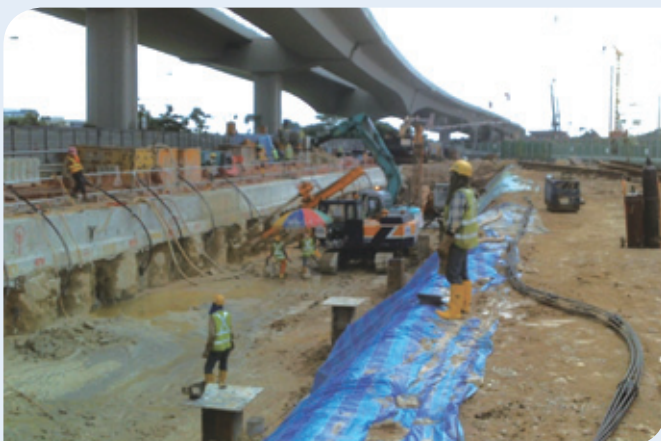
Figure 5: Installation of ground anchors
