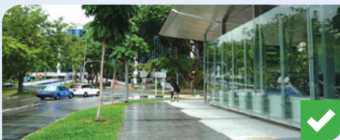
Figure 7: Adequate offset of station structure from road edge
