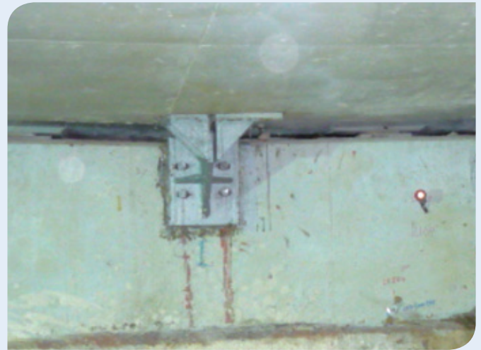
Figure 2: Additional lateral steel bracket installed to the abutments
