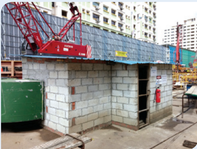
Figure 1: Noise Enclosure for Ventilation Fan
