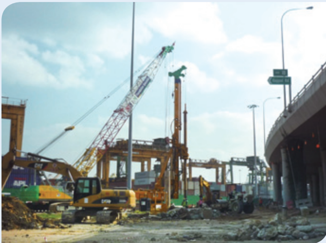
Figure 4: Piling works beside flyover
