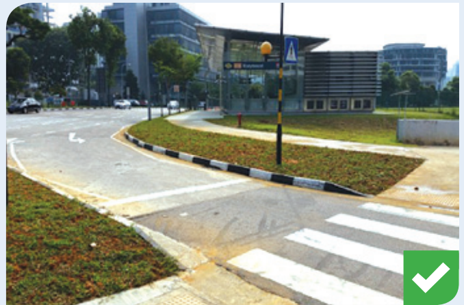
Figure 4: Station entrance located away from slip road of junction provides good view of pedestrian at crossing point
