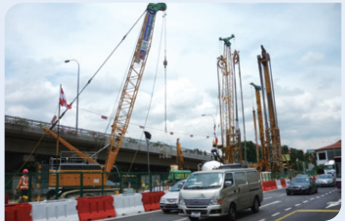
Figure 6: Lifting works beside flyover
