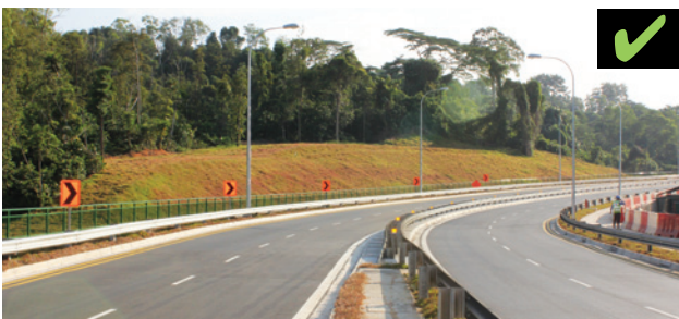
Figure 2: Crossfall and longitudinal gradient are required along the carriageway to channel the surface runoff to the roadside drains.
