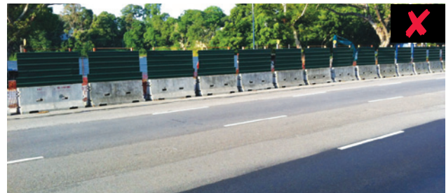
Figure 5: The precast concrete safety barrier segments have been disconnected to create gaps to allow surface runoff to flow towards the roadside drain. However, while this may address the drainage issue, the precast concrete safety barrier will no longer be able to serve its function as a safety barrier and will create undue roadside safety issues.
