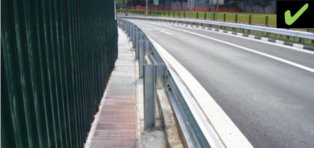
Figure 8: Use of a drain covered with vehicular grating behind the w-beam guardrail which will also allow for the dynamic deflection of the w-beam guardrail when impacted.
