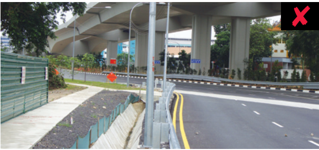
Figure 7: If the w-beam guardrail is impacted, the impacting vehicle is likely to crash into the open drain as the w-beam will not be able to cater for the vehicular impact. This is due to insufficient space behind the guardrail for it to deflect in order to safely contain and redirect the vehicle back onto the carriageway.
