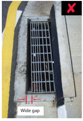
Figure 10: Improper construction of drainage inlets with wide gaps along the carriageway could pose stability problems for cyclists.
