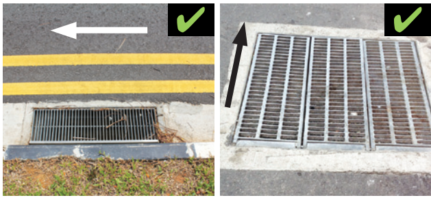
Figure 11: The current design standards require the provision of drainage inlets with gratings that are perpendicular to the direction of travel and smaller gaps in-between the gratings.
