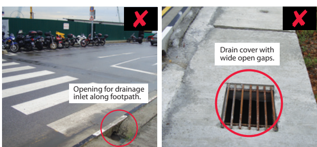
Figure 9: Improper surface openings for drainage inlets along the footpath will create a tripping hazard for pedestrians.
