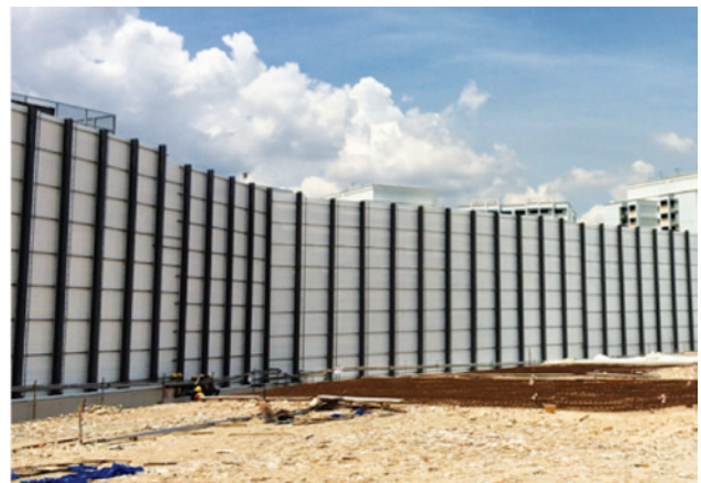
Figure 3: Erection of 10m noise barriers on the side facing noise sensitive receptors
