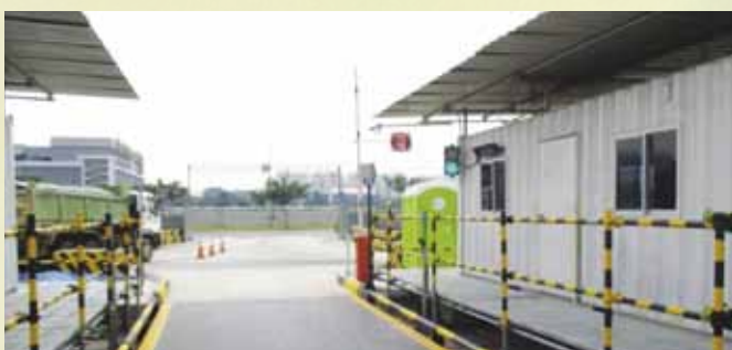
Figure 7: Workers are not exposed to vehicular movements
