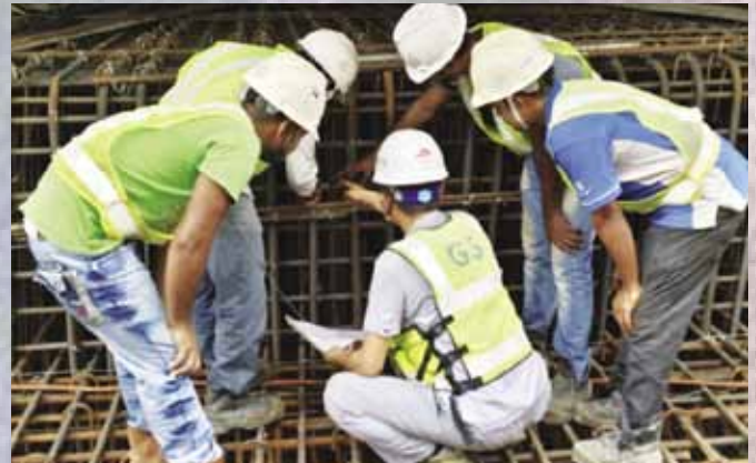
Figure 1: On the job trainings conducted on site to increase the skill level of workers
