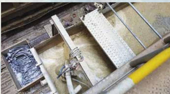
Figure 4: Separate containment of tunnelling wastewater at the bottom of the launch shaft
