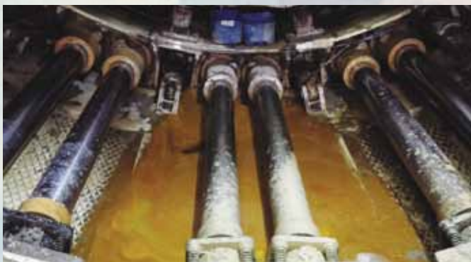
Figure 3: Hydraulic oil spillage at cutter head
