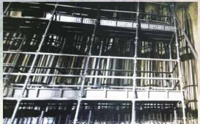
Figure 2: Scaffold erected by a team of formwork erectors that are competent in scaffold erection
