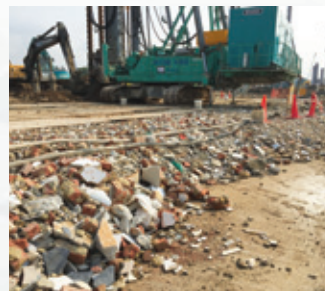
Figure 7: Industrial debris used as hardcore material
