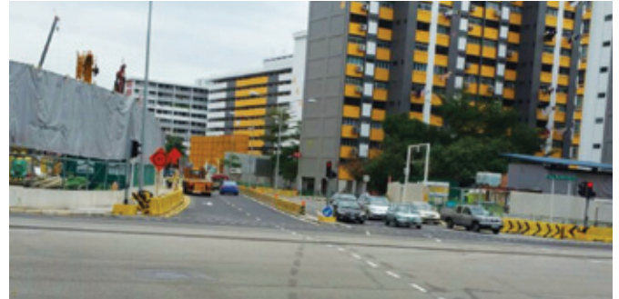
Figure 7: Improved alignment across the junction in subsequent stage of diversion
