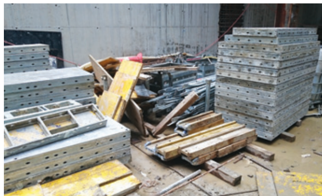
Figure 6: Excess material within the station box
