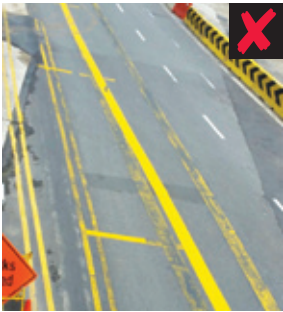
Figure 3: Obsolete pavement markings overlapped with new pavement markings
