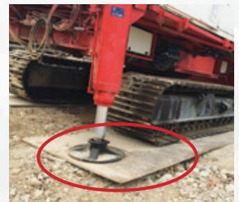
Figure 8: Working platform not properly compacted resulting in voids beneath steel plate
