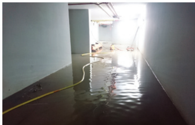
Figure 7: Water stagnation on slab
