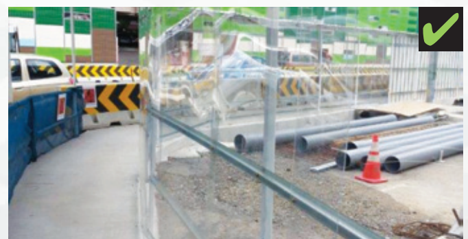
Figure 2: Clear view at the corner of the junction with acrylic panels
