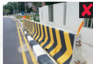
Figure 9a: Improper placement of concrete barriers on kerb
