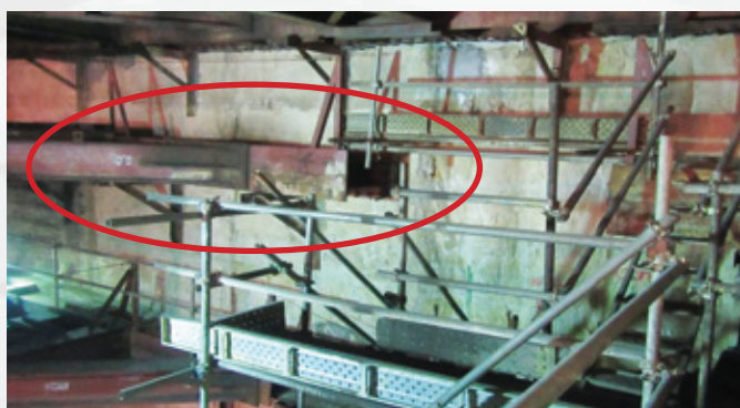
Figure 5: An intermediate level waler
