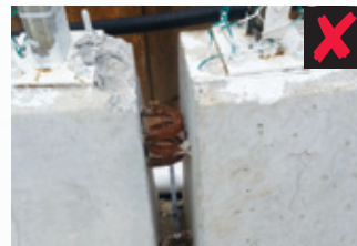
Figure 8a: Missing interlocking pin between the concrete barriers
