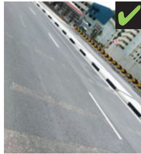
Figure 4: Obsolete pavement markings have been milled off
