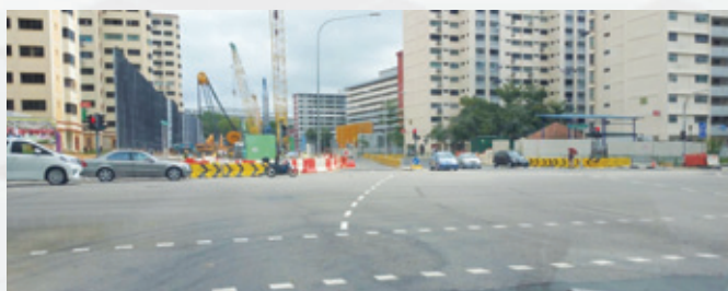
Figure 6: Guidelines provided across misaligned junction
