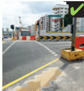
Figure 5b: Unobstructed crossing point provided
