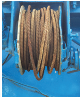
Figure 5: Inadequate greasing leading to corrosion of wire ropes
