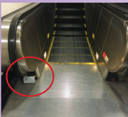
Figures 2 : Location of speaker device installed on escalators
