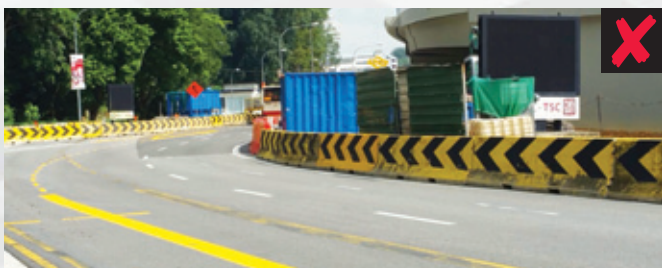
Figure 1: Container placed within the line of sight around inner road bend
