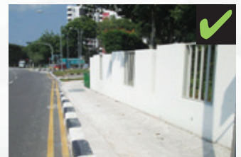
Figure 9b: Removal of concrete barrier on kerb after rectification
