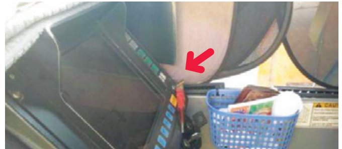
Figure 6: Key to the bypass switch inserted in the control panel
