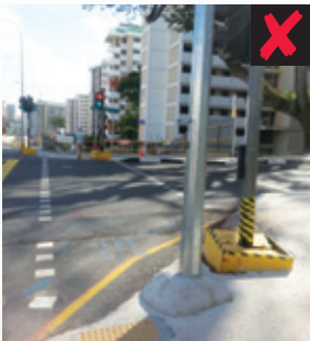
Figure 5a: Obstruction in the middle of crossing point
