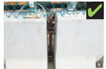
Figure 8b: Interlocking pin installed between the concrete barriers
