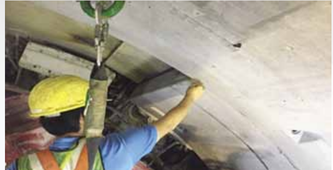
Figure 4: Measures for Work at Height in place
