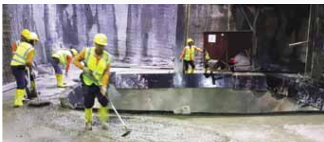
Figure 3: Concrete casting of basement at facility building
