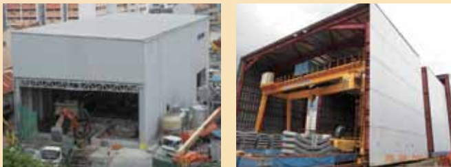
Figure 5: Full noise enclosure at DTL C935 (left), and retractable noise enclosure at TEL T216 (right) installed at launch shafts for noisy tunnelling works
