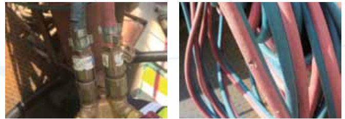
Figure 8: Damaged / cracked gas hoses
