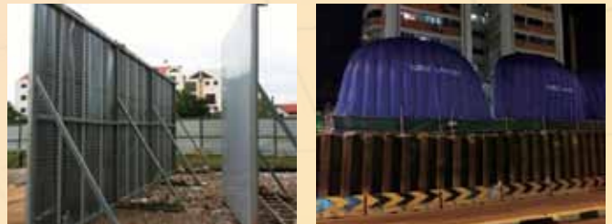
Figure 7: Mobile noise barrier at DTL C923 (left) and air inflated temporary noise barrier at TEL T211 (right)
