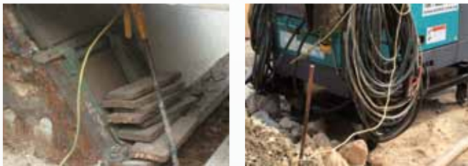
Figure 5: Welding machines not adequately earthed
