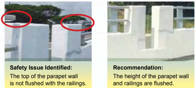
Figure 2d: Safety issue identified before public opening of a new road after completion
