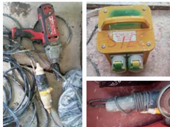
Figure 9: Electrical equipment / tool without LEW's monthly inspection sticker
