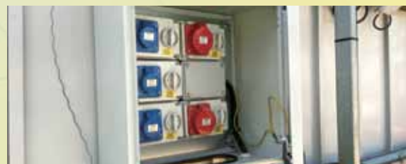
Figure 4: SOA with weatherproof box cover
