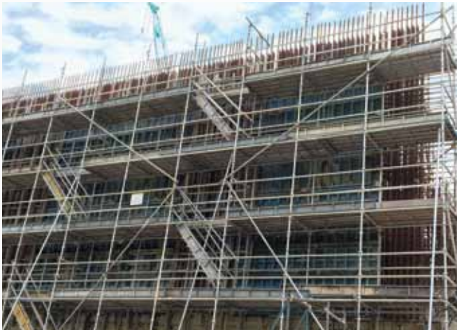
Figure 5: Example of good edge protection where guardrails and toe boards are securely installed
