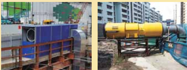
Figure 6: Noise enclosure over the ventilation fan unit at TEL T221 (left), and ventilation fan silencer installed at DTL C929A (right)
