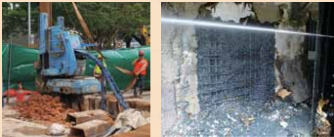
Figure 4: Use of a silent piler (left) and aqua cutter (right)
