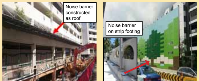
Figure 8: Noise panels was used to construct roof canopy at TEL T211 along the corridor (left), and noise barrier was constructed on a narrow strip footing at TEL T216 to overcome space constraint (right)
