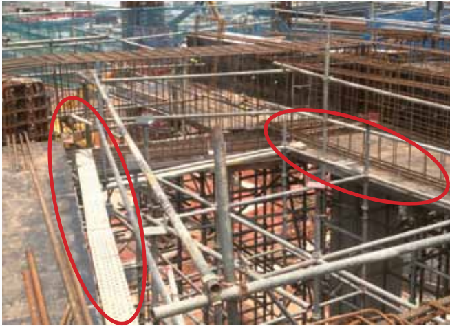
Figure 4: Example of poor edge protection where there is risk of person falling from open sides
