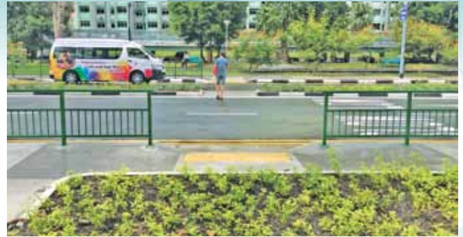
Figure 6: Kerb-cut ramp with railings and landscaping along Lorong 8 Toa Payoh
