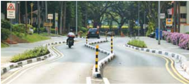
Figure 4: Chicane along Bukit Merah View (top); 2-to-1 lane Pinch Point along Marine Terrace (bottom)
