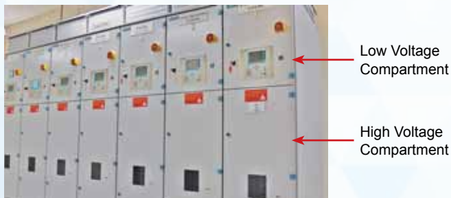
Figure 2: A typical DC Switchgear inside a Traction Power Substation
