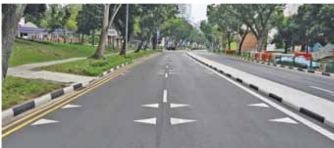
Figure 5: Traffic Calming Markings along Bedok North Street 1
