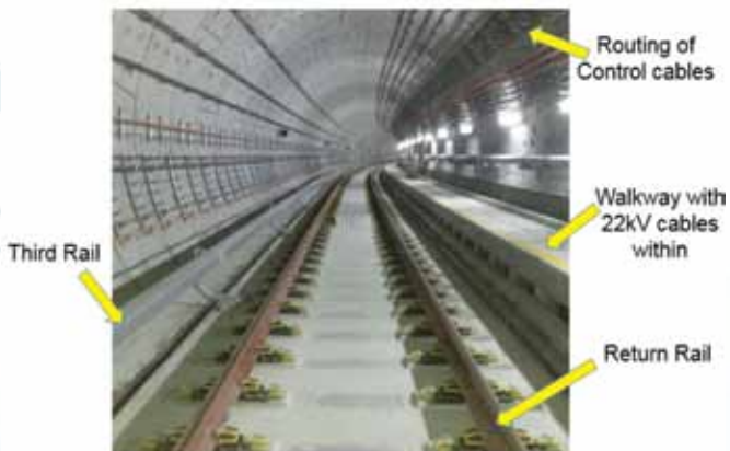
Figure 1: Third Rail System in a tunnel
