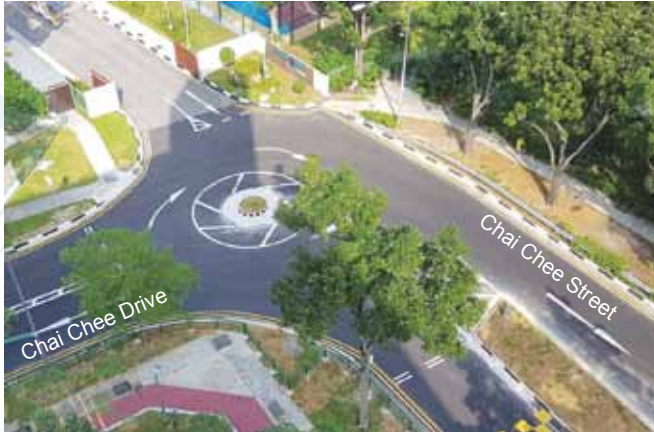
Figure 1: New roundabout at Chai Chee Street / Chai Chee Drive junction
