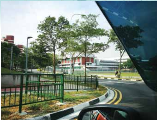
Figure 4: A driver's view after the implementation of a roundabout. The new single lane roundabout eliminates obstruction caused by vehicles, giving drivers a clear line of sight
