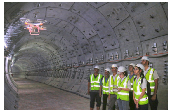
SUBTERRANEAN INSPECTION LTA officers are piloting the use of drones to monitor new tunnel constructions.
