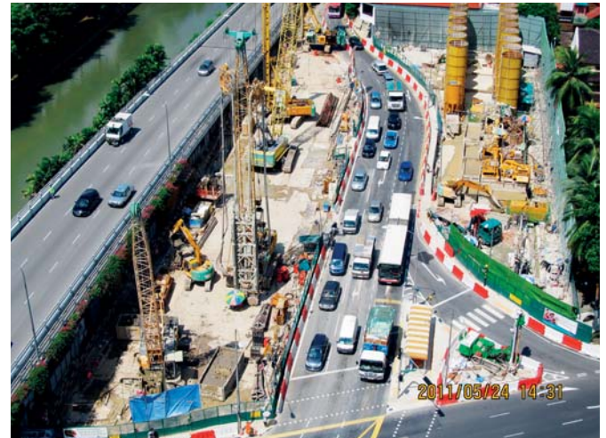
Figure 10: Completion of road diversion
