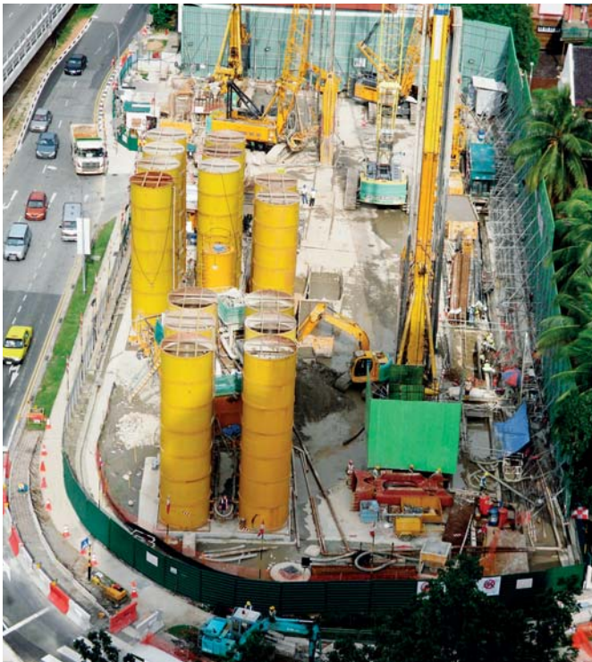
Figure 6: Space constraint on site
