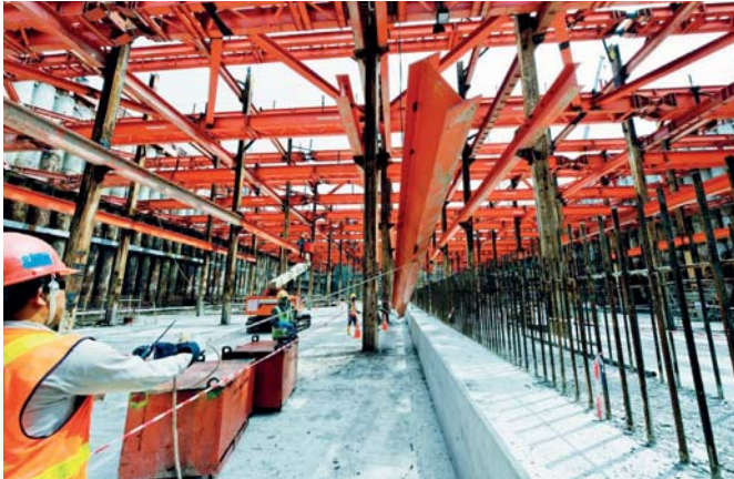
Figure 5: Use of tag line to control the load
