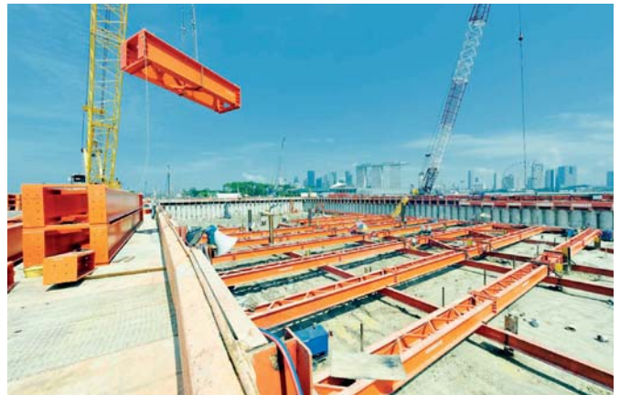
Figure 4: Ensure that workers are not required to work under suspended loads
