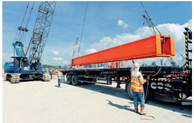
Figure 3: Crane setup on firm ground and level surface
