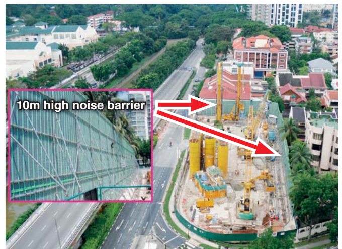
Figure 4: Erecting noise barrier around the worksite
