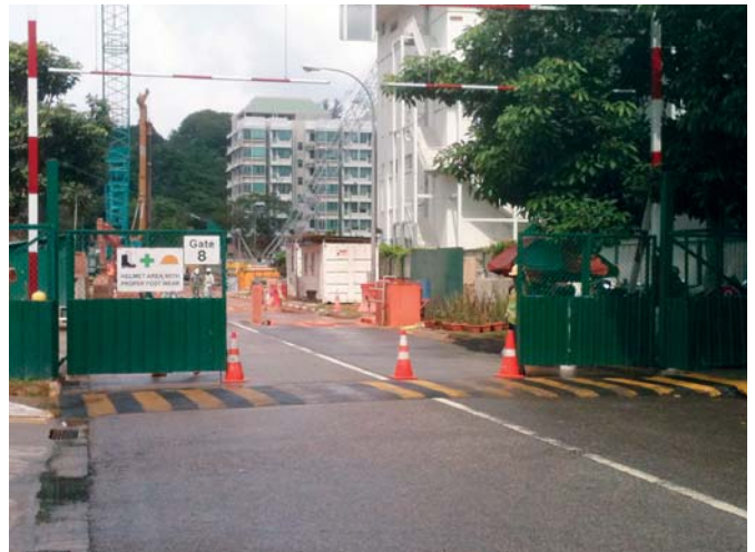
Figure 2: Site access arrangement at high pedestrian movements area
