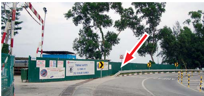
Figure 4: Proper end treatment of VIG
