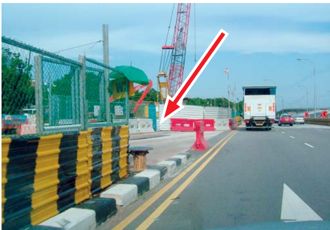
Figure 1: Lay-by with acceleration lane
