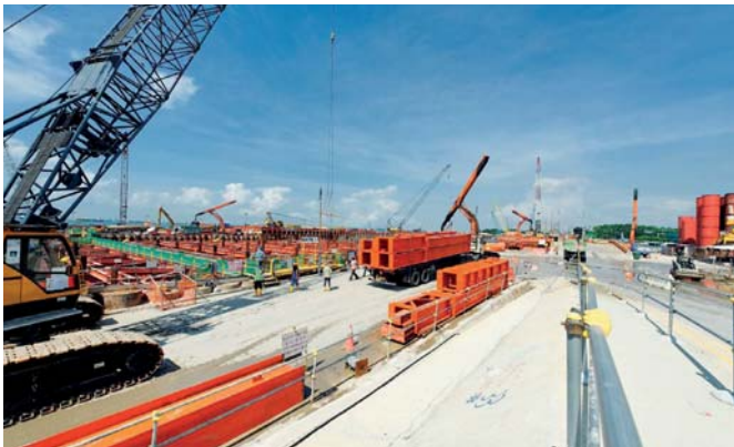
Figure 2: Adequate access route to ensure safe delivery and movement of machinery and materials
