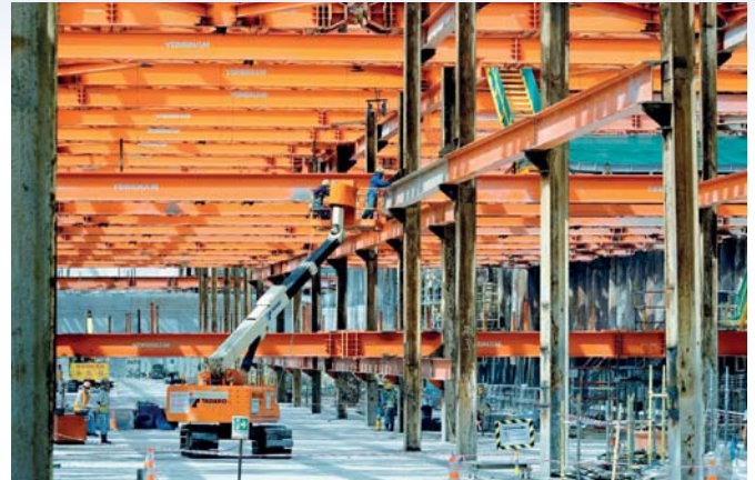
Figure 7: Use of boom lift as an alternative for working at height
