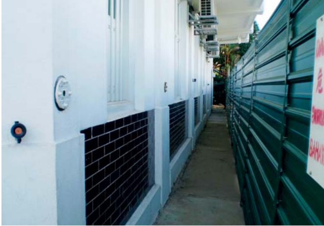
Figure 5: Ensuring adequate walkway/access spaces
