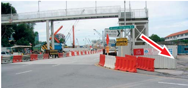
Figure 3: Poor site access arrangement near junction
