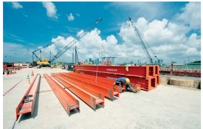
Figure 8: Proper storage of materials and maintain good housekeeping at work site
