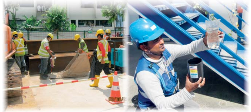
Carpet combing exercises aimed at eradicating potential breeding grounds were carried out at LTA construction sites
