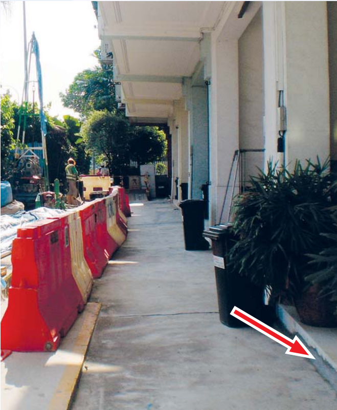
Figure 8: Settlement of the nearby shophouses (patched up with cement)
