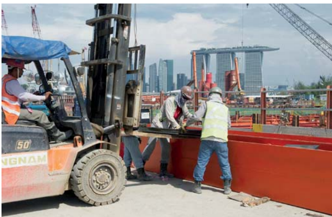
Figure 6: Appropriate machinery to help worker handle heavy or irregularly-shaped loads
