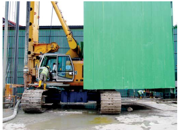
Figure 3: Noise barriers installed to contain noise
