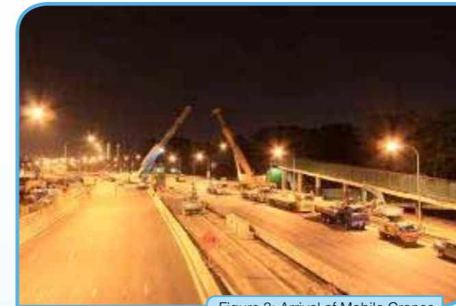
Figure 3: Arrival of Mobile Cranes
