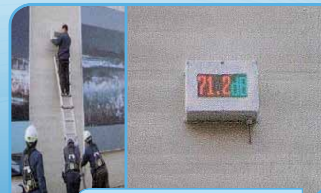
Figure 4: Installation of display box for the monitoring of construction noise
