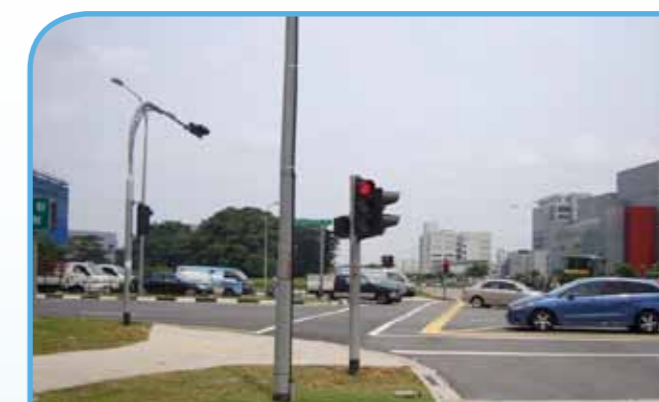
Figure 10: Proper coordination in the placement of the street furniture to ensure that the street light pole is located sufficiently away from the carriageway so that it does not obscure the visibility of the traffic signal
