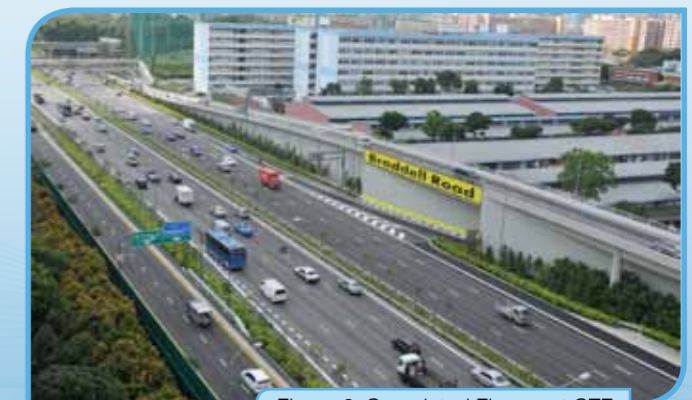
Figure 6: Completed Flyover at CTE
