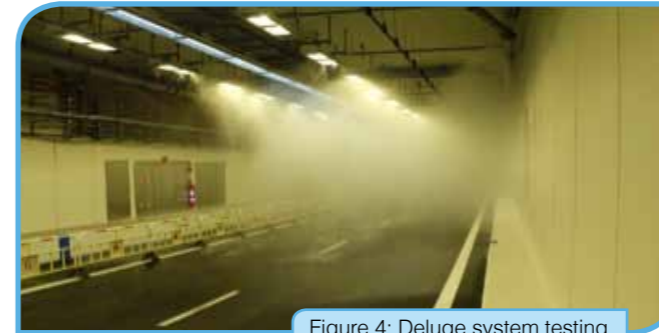
Figure 4: Deluge system testing
