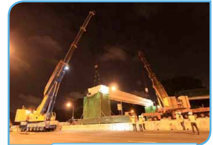
Figure 5: Completion of PSPC Beam Launching
