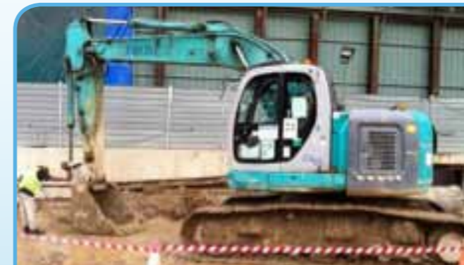
Figure 7: Excavator operator conducting pre-operation checks
