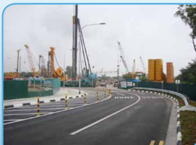
Figure 5: At work zones, site hoardings installed across the road bend, rather than along the inner radius
