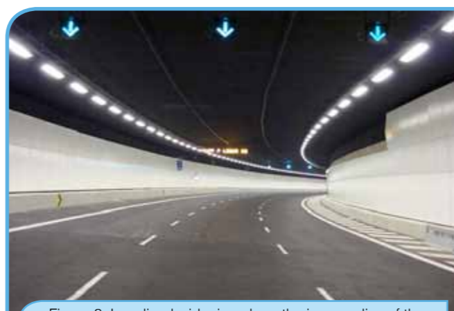
Figure 3: Localised widening along the inner radius of the road bend to provide a wider offset between the carriageway and the tunnel structure
