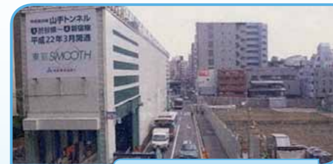
Figure 3: Total noise enclosure in Japan
