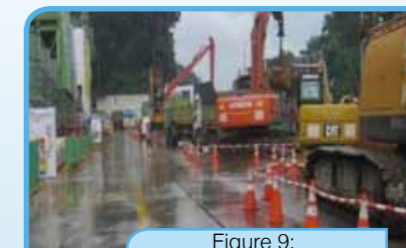
Figure 9: Work area cordoned off
