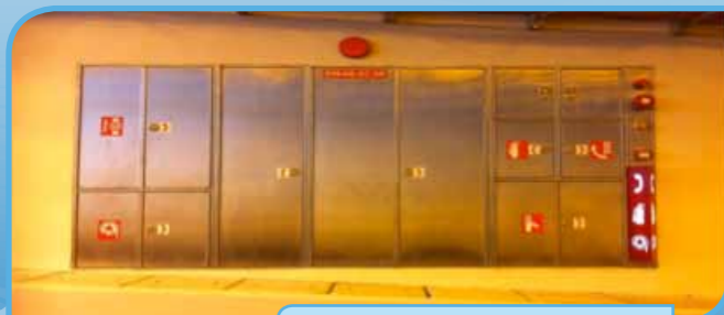
Figure 2: Emergency niche at WVT
