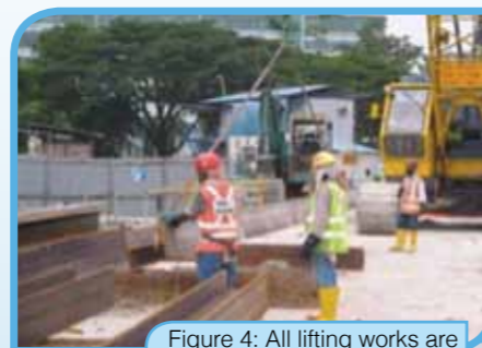
Figure 4: All lifting works are closely supervised
