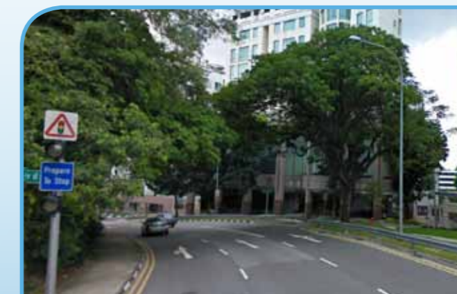
Figure 11: Advanced Warning Lights (AWL) provided to alert motorists about the signalised traffic junction after the road bend
