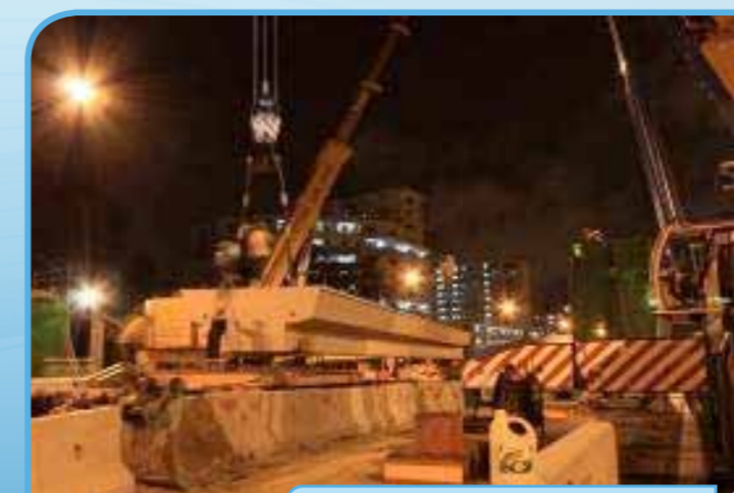
Figure 4: Hooking up of PSPC Beams
