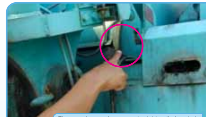
Figure 6: Inspection: over-derricking limit switch
