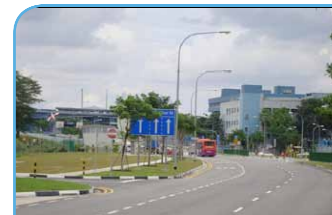
Figure 9: The presence of trees too close to traffic sign would obscure visibility. Based on LTA Design Criteria, trees are to be planted at a minimum distance of 45m and 75m away from advanced directional signs for non-expressways and expressways respectively
