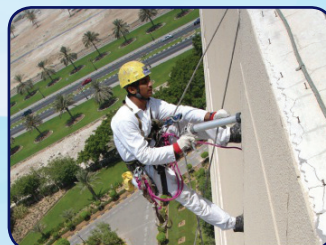
Figure 5: Use of industrial rope access equipment 1
