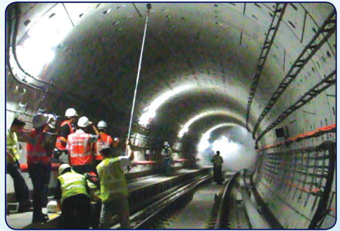
Figure 5: Smoke tests conducted to verify effectiveness of tunnel ventilation system during testing & commissioning
