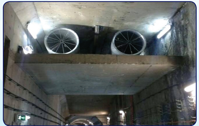
Figure 2: Tunnel booster fans installed in tunnels
