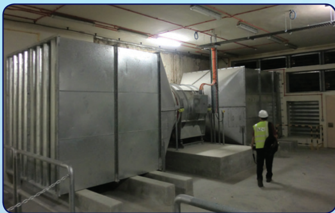
Figure 1: Tunnel ventilation fan room
