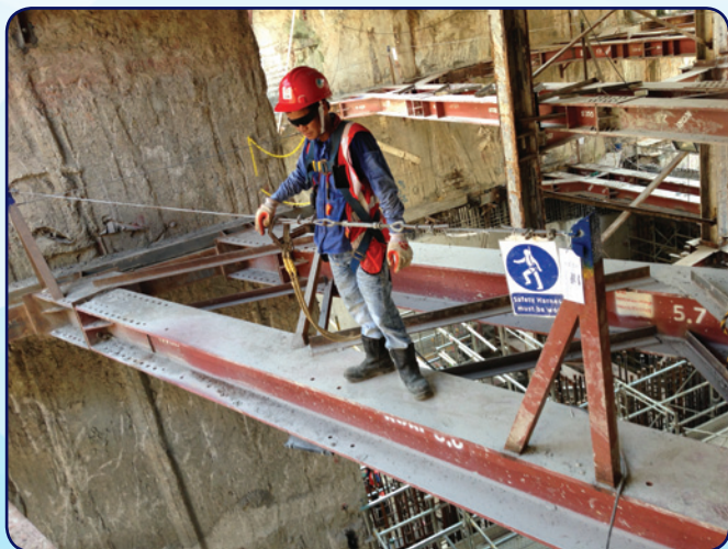
Figure 4: Use of fall arrest system
