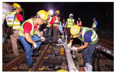
Third rail replacement works were carried out on the North-South Line for a more reliable train network. Extended engineering hours allow for renewal works to be completed faster.
