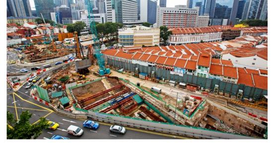
Bulk excavation and casting work carried out at the upcoming Maxwell station along the Thomson-East Coast Line.
