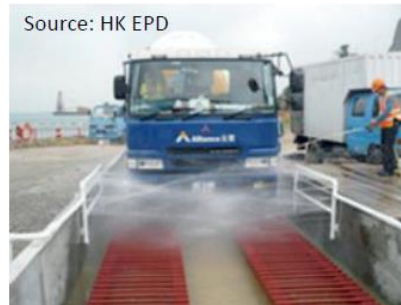
Vehicle washing facilities at exit point from construction site
