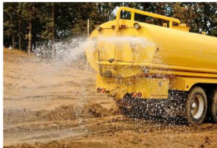
Dampen construction site with water regularly
