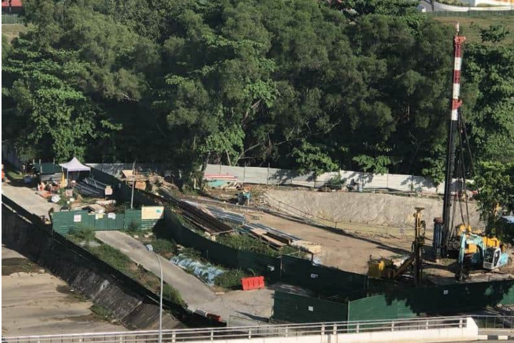
Figure 3-7 Example of slope cutting works [O-5]
