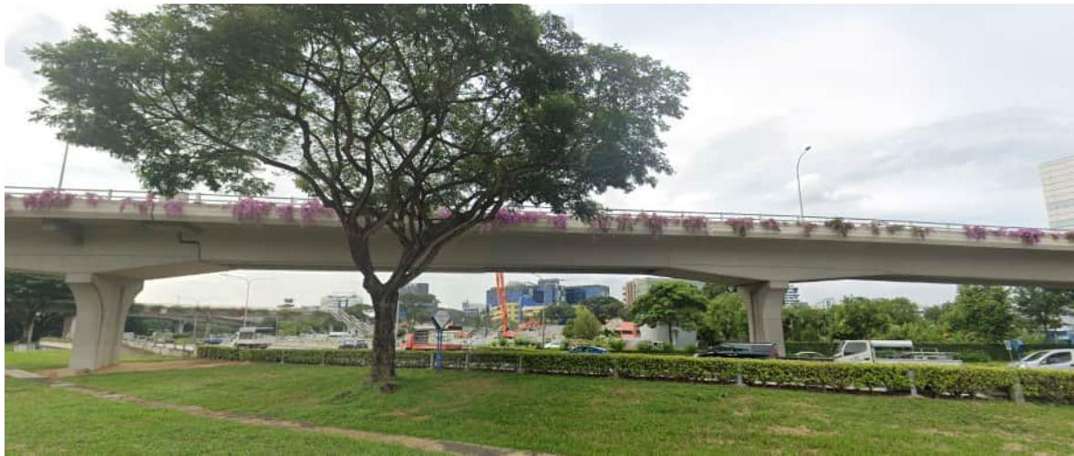
Figure 3-23 Example of pre-cast U-beam with cast-in-situ RC columns of Aljunied West Flyover
