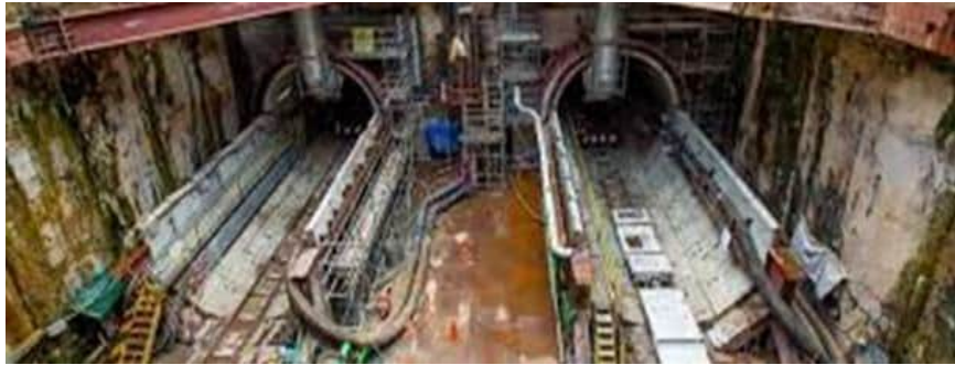
Figure 3-12 Example of slurry TBM [W-22] and twin-bored tunnel at a station site in Singapore [W-23]
