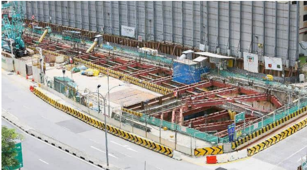
Figure 3-18 Example of construction site employing top-down construction method [W-18]
