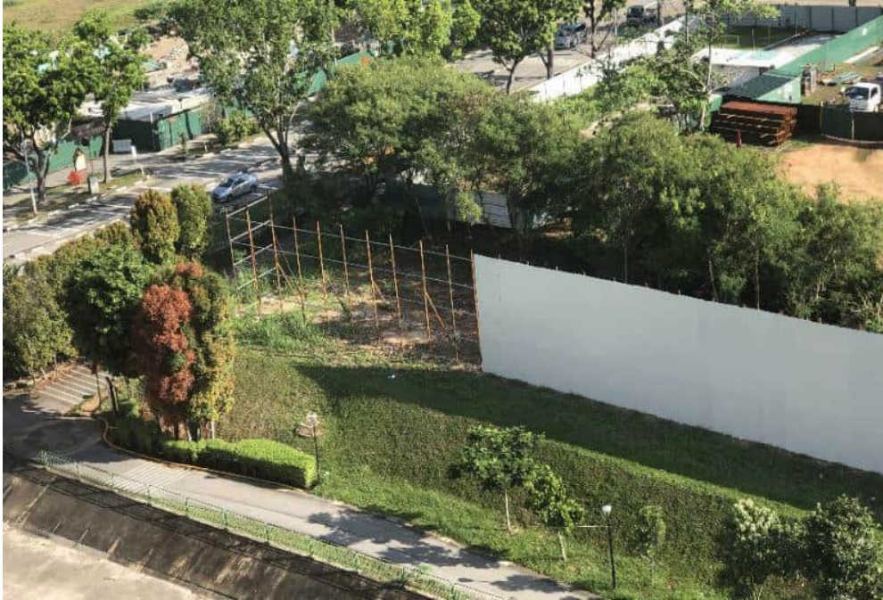
Figure 3-5 Example of site hoarding erection [O-5]
